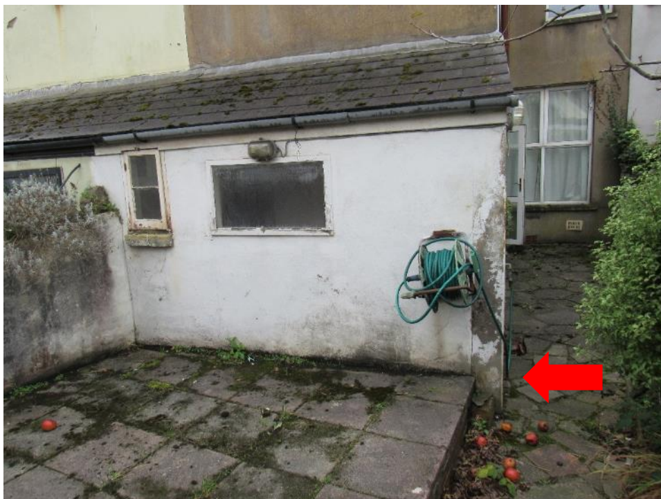
Photograph 52: External view of the downstairs toilet/utility room (note height of patio)
