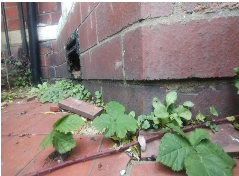
Photograph 16: Bay window – historic oversailing (mortar original/good condition)
