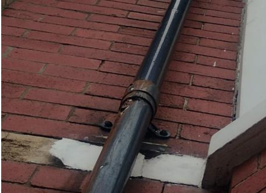
Photograph 13: Drainage – replacement of front downpipe required
