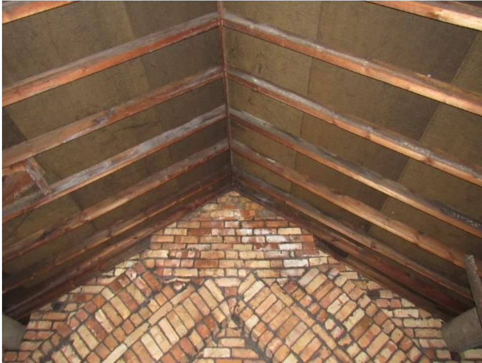
Photograph 37: Roof internal – ridge board in fair condition
