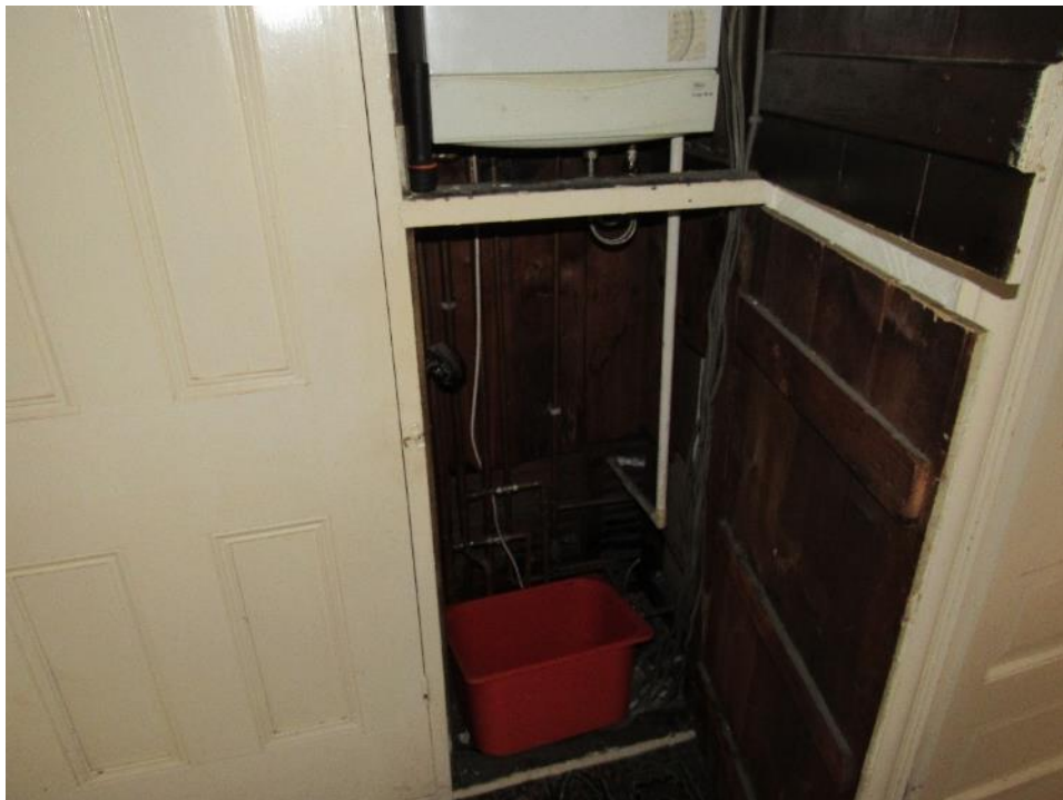
Photograph 70: Boiler – possible active leak
