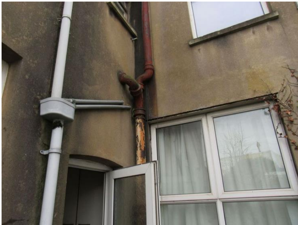
Photograph 12: Soil pipe – cast iron
