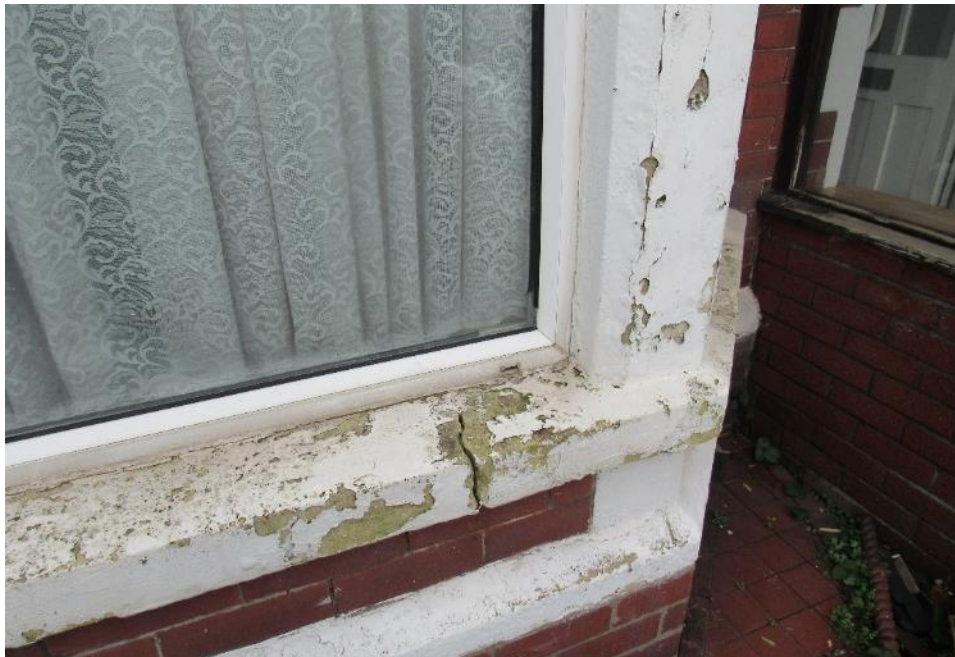
Photograph 14: Bay window – fracture to lower sill
