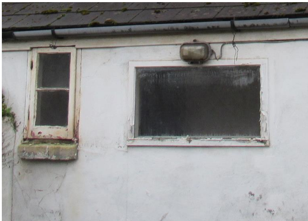
Photograph 30: Windows/doors – single pane units
