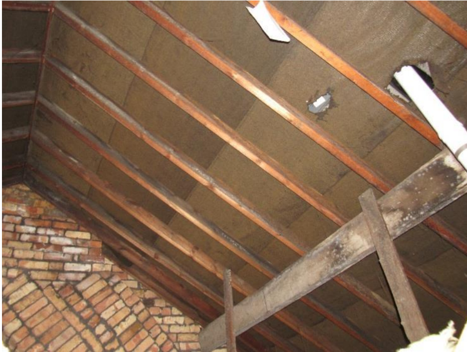
Photograph 39: Roof internal – sarking mostly in fair condition, isolated patch repairs noted
