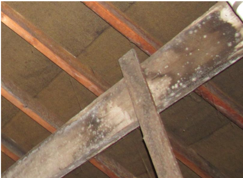
Photograph 38: Mould growth/damp to purlins
