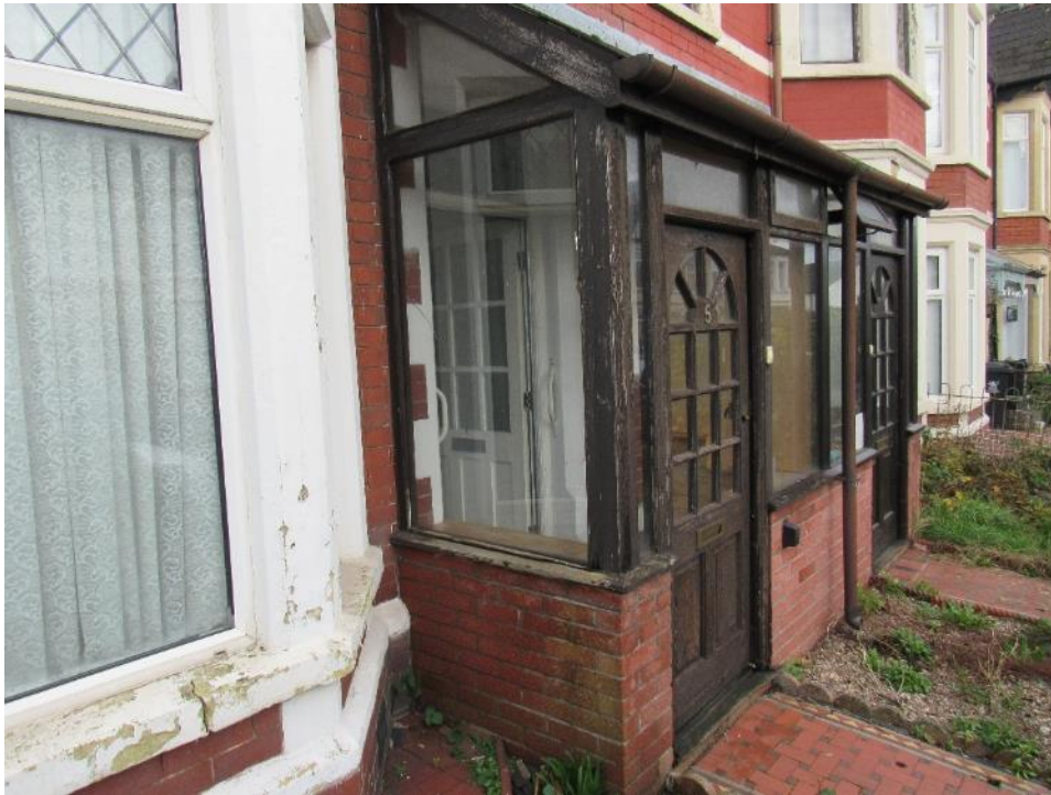
Photograph 35: Porch – wooden elements in poor condition
