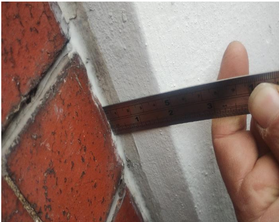
Photograph 18: Bay window – no significant movement to jambs noted
