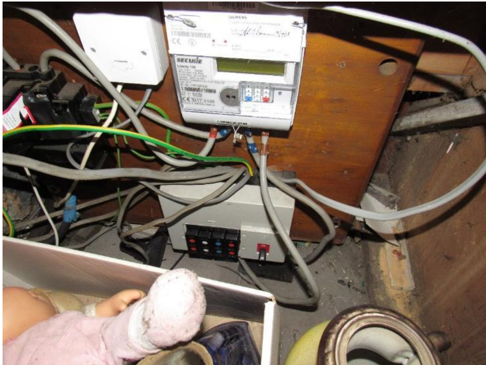
Photograph 68: Electrical – consumer unit (fuse board) under the stairs
