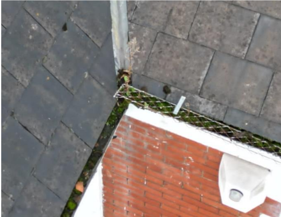
Photograph 9: Gutters – moss/blockages
