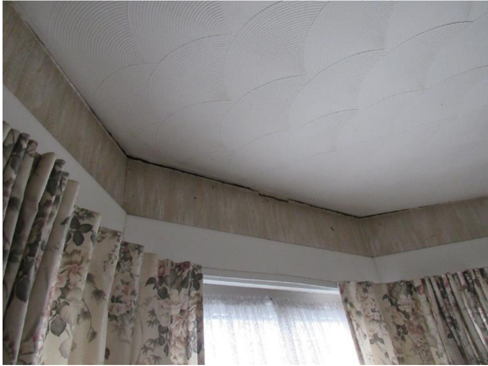
Photograph 21: Bay window - internal view/fracture to upper
