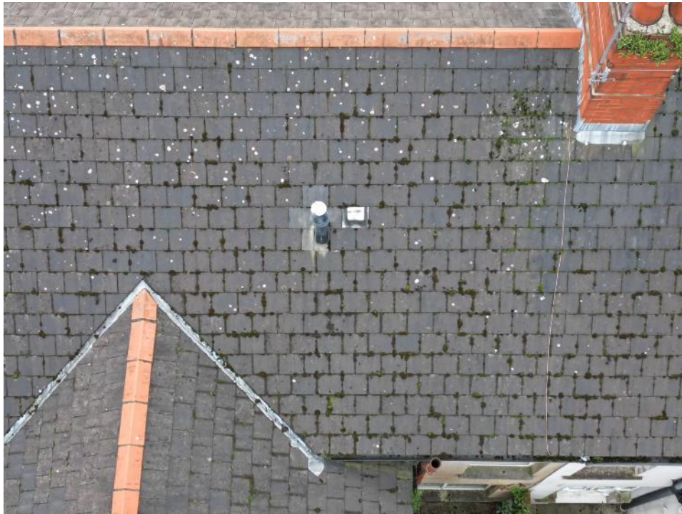
Photograph 7: Roof – rear pitch condition (note moss growth)
