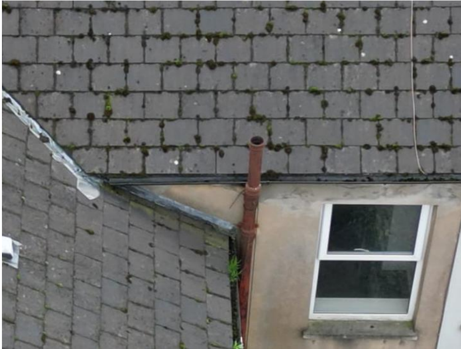
Photograph 11: Soil pipe – cast iron
