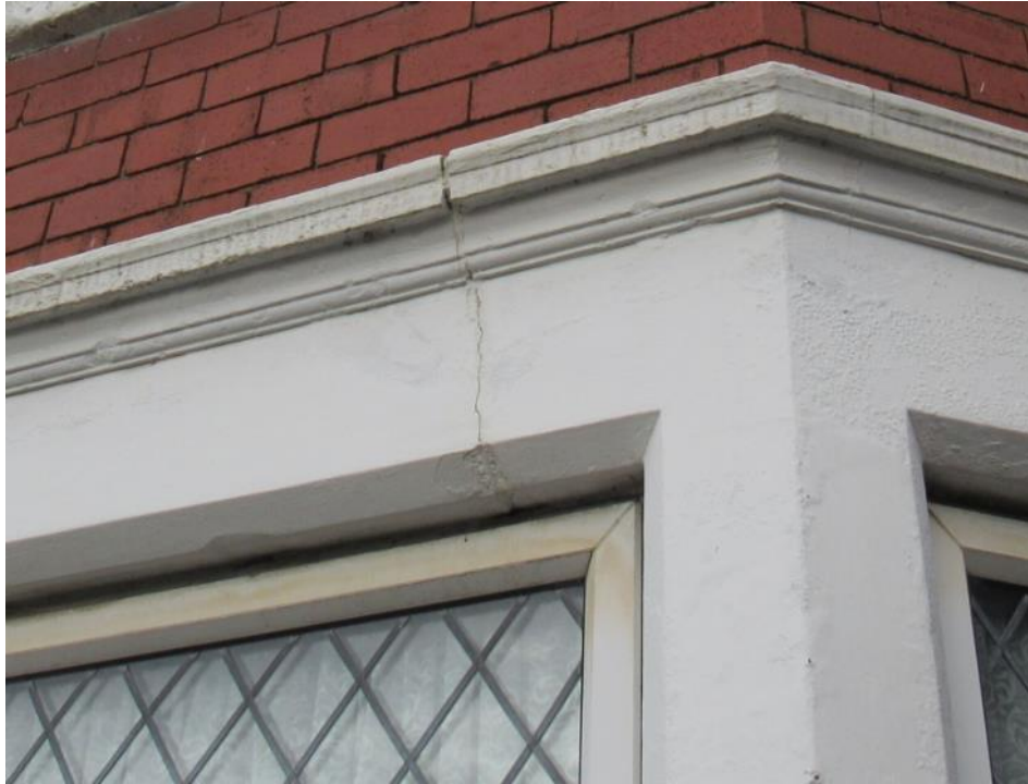
Photograph 15: Bay window – fracture to upper sill
