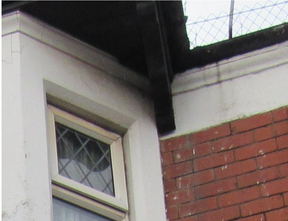
Photograph 23: External walls – corbel displaced (note shadow)
