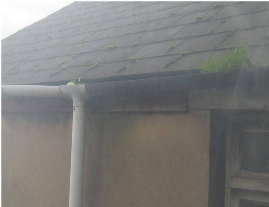
Photograph 10: Gutters – moss/blockages
