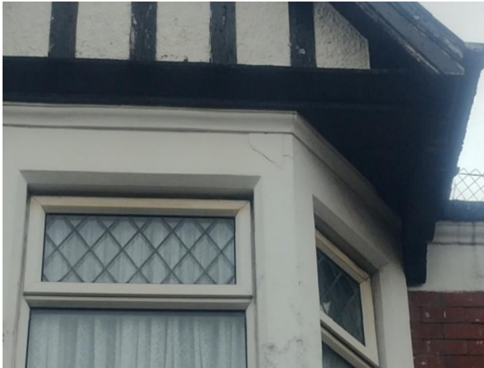
Photograph 19: Bay window – fracture area to upper
