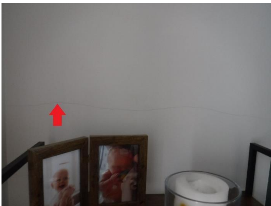
Photograph 32: Hairline plaster crack to dining room adjacent to chimney stack
