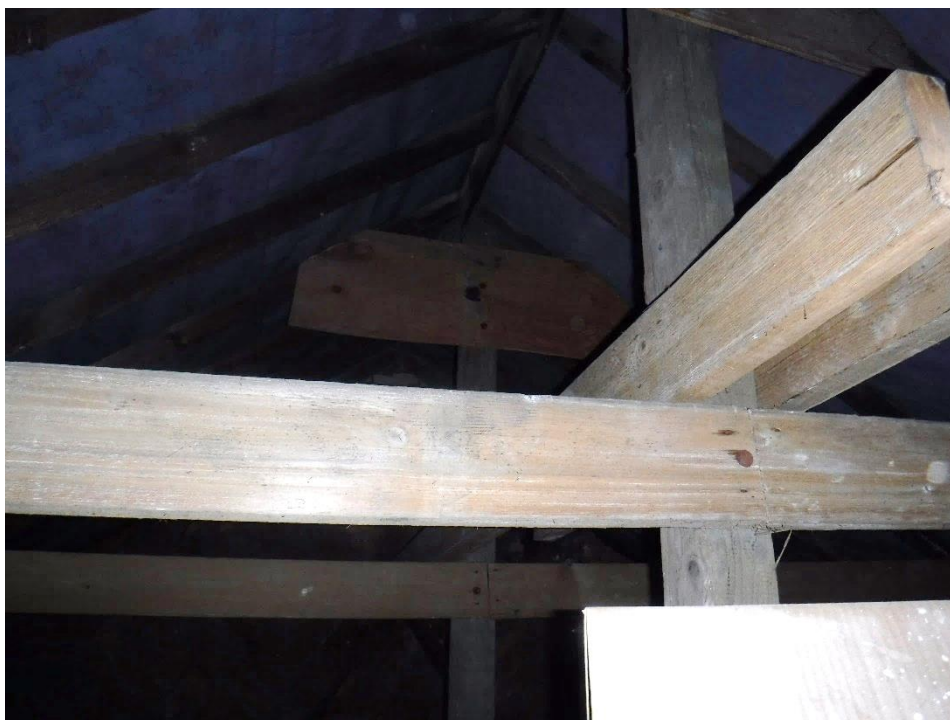
Photograph 22: Roof space - Kingpost located centrally
