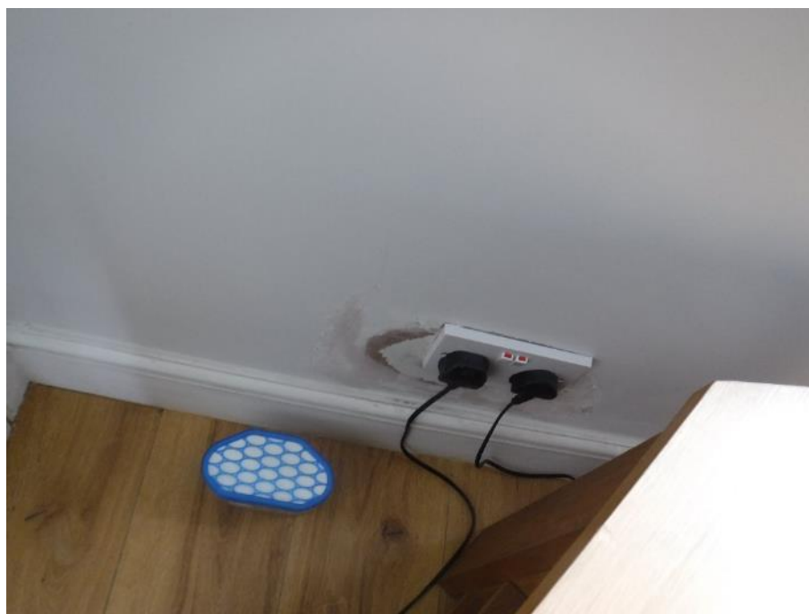
Photograph 30: A small damp patch was noted in the sitting room on the SW corner
