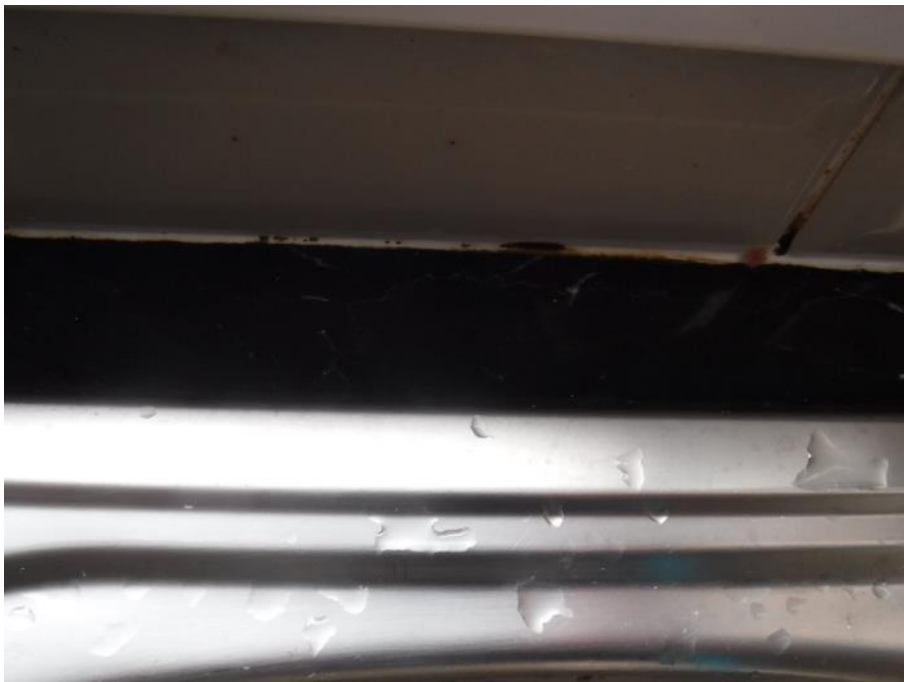
Photograph 44: Minor sealant repair around some of the tiled areas in the kitchen area
