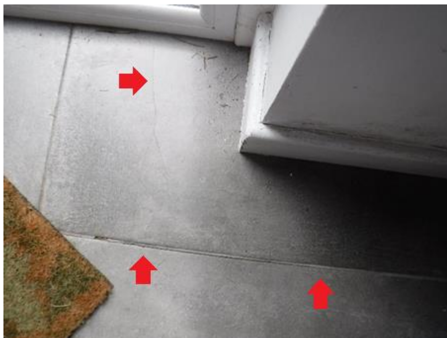
Photograph 38: Kitchen – cracks noted to single tile
