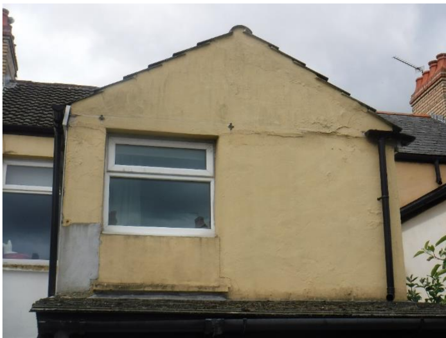
Photograph 12: Rear elevation – render repair required
