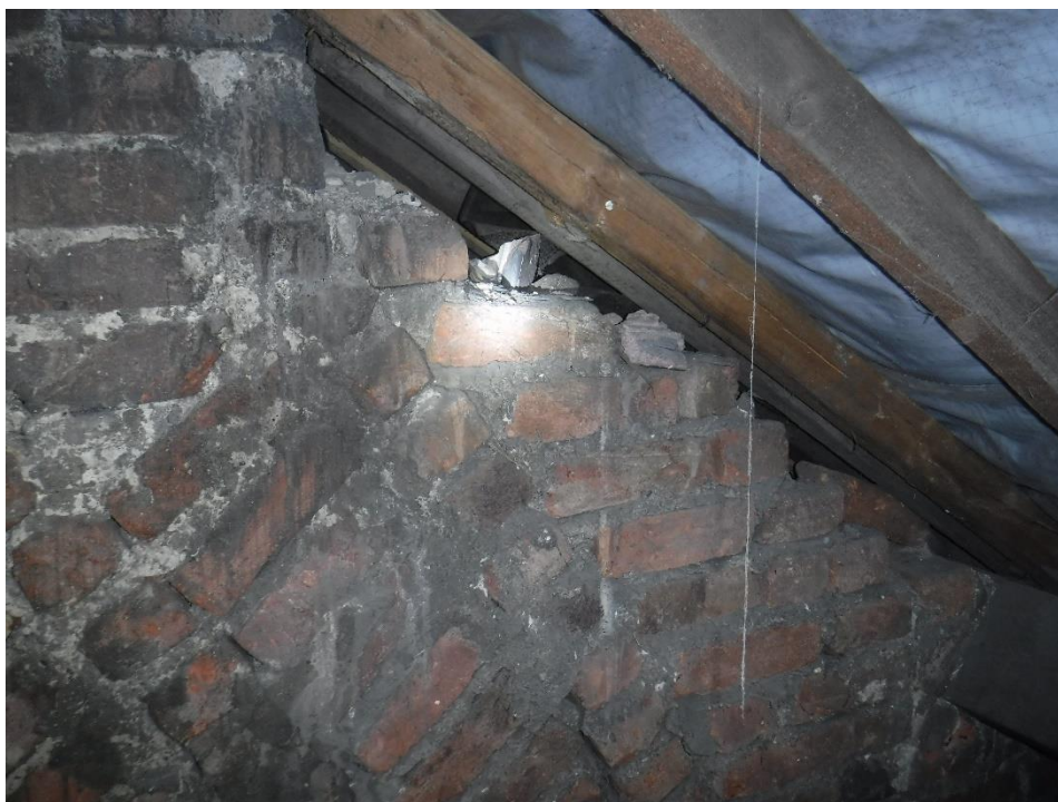
Photograph 20: Roof space - Lack of fireproofing up to top
