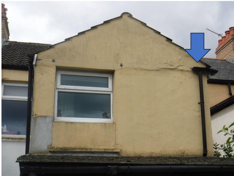
Photograph 7: Rear projection - downpipe dispels onto bathroom roof...
