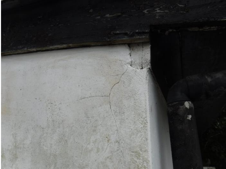
Photograph 13: Bathroom extension high level – hairline crack
