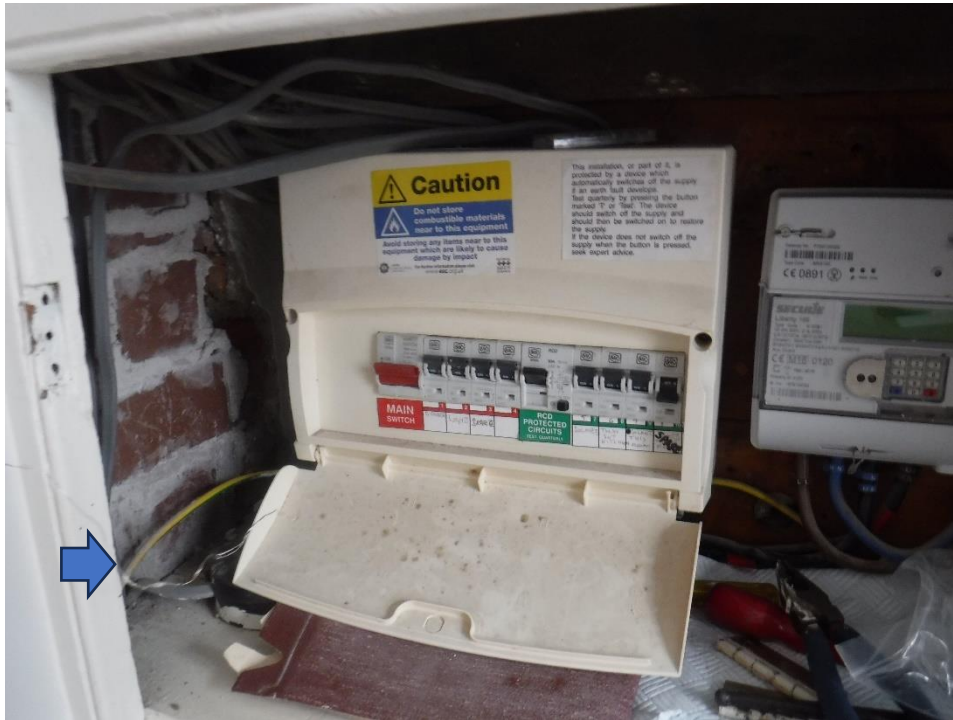
Photograph 49: Consumer unit (note stray wire)
