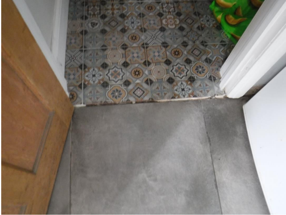
Photograph 35: Floors - missing threshold
