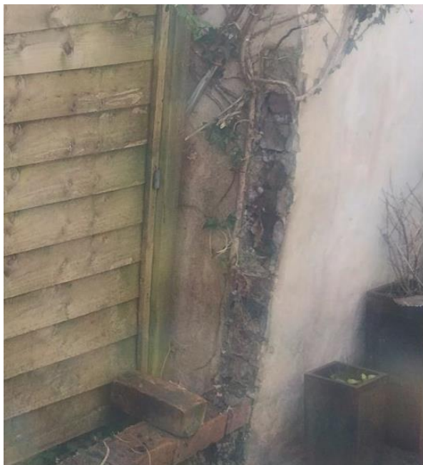
Photograph 63: Extension bulge - contrasting the existing quoin with a typical keyed corner (quoin)
