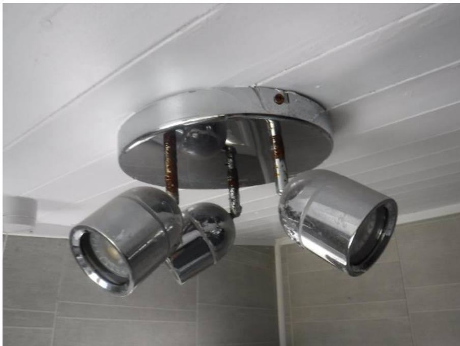
Photograph 47: Surface corrosion to light-fitting in bathroom
