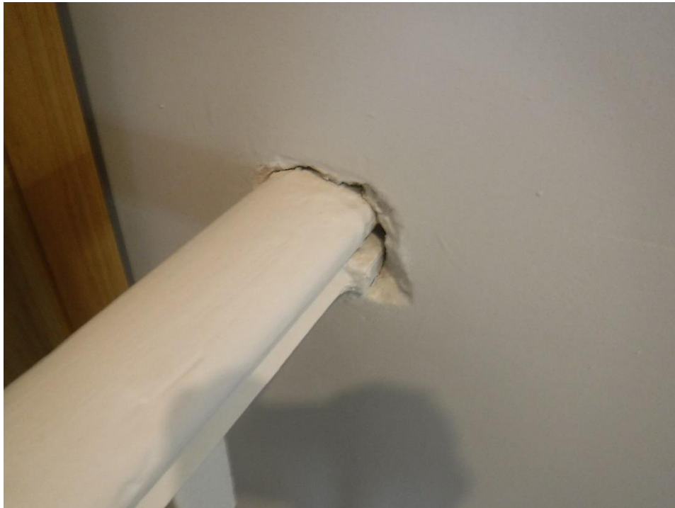
Photograph 46: Balustrade interface – plaster breakdown
