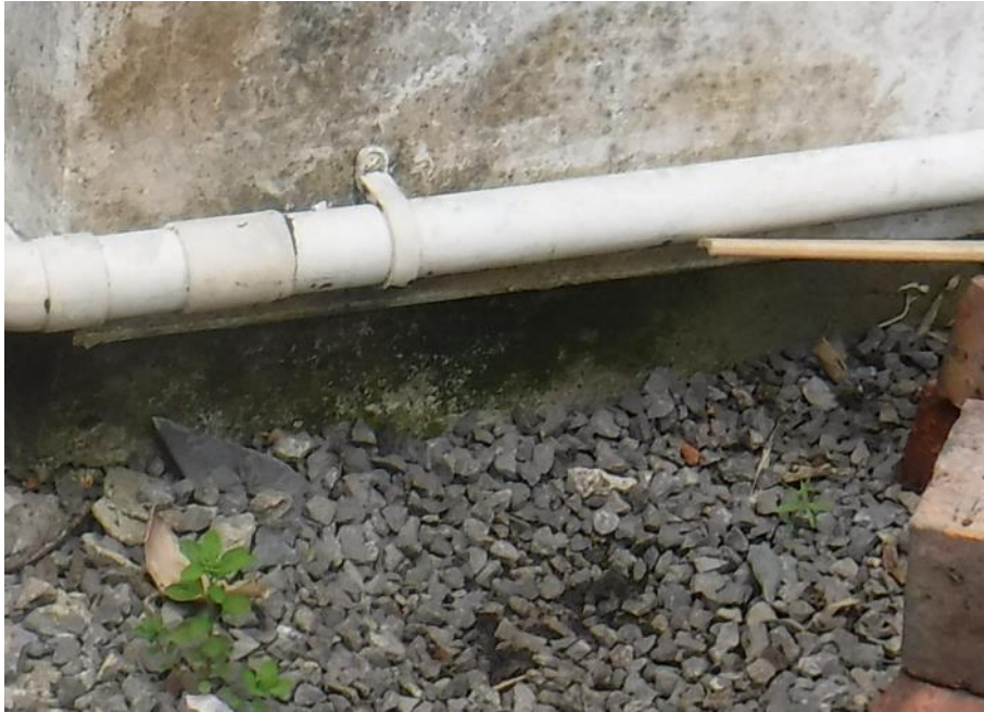
Photograph 15: Bathroom extension - the render extends to ground level possibly bridging DPCs
