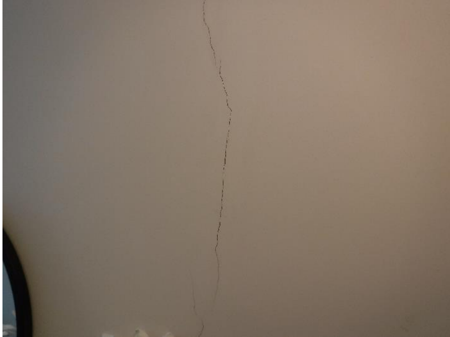
Photograph 33: Hallway – vertical 1-2mm crack
