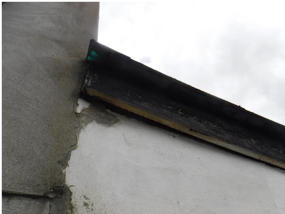
Photograph 17: The fascias require updating or treating
