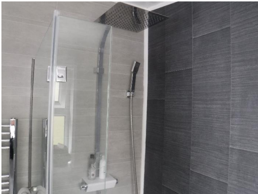
Photograph 34: PVC bathroom panels to bathroom
