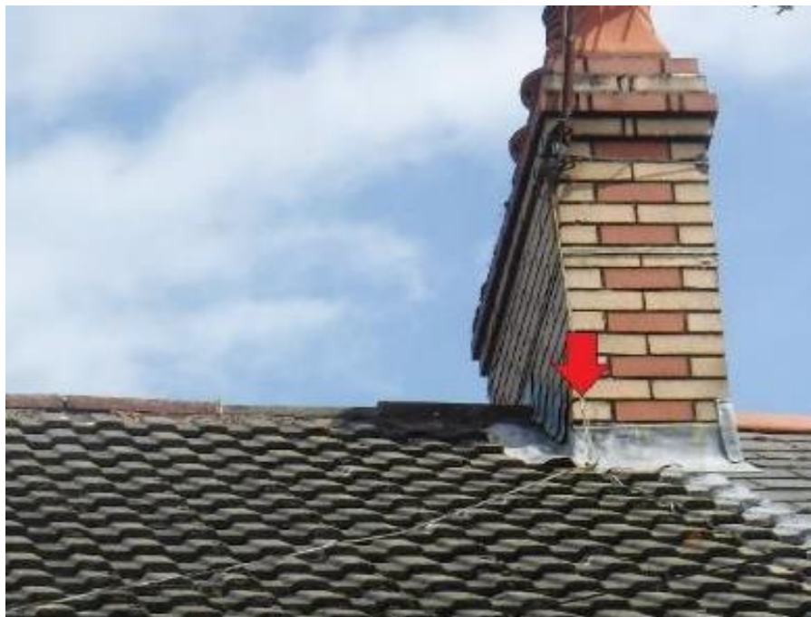
Photograph 3: Chimney – corner flashing at base missing
