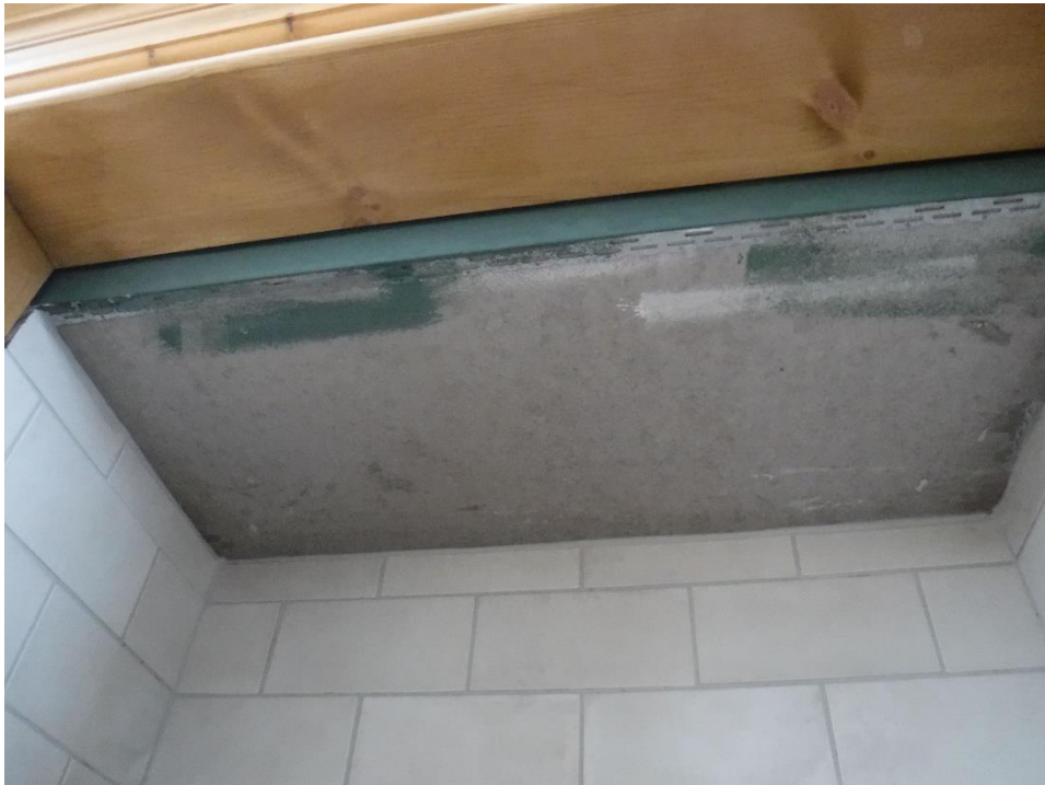
Photograph 42: Chimney breast boxed off
