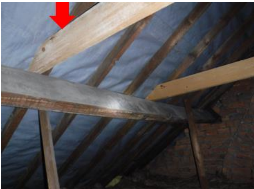
Photograph 23: Roof space - Kingpost horizontal members
