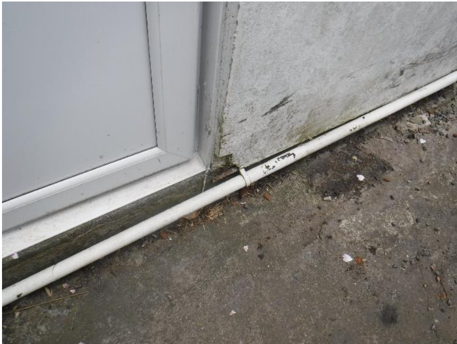
Photograph 14: Kitchen door low level – patch render repair
