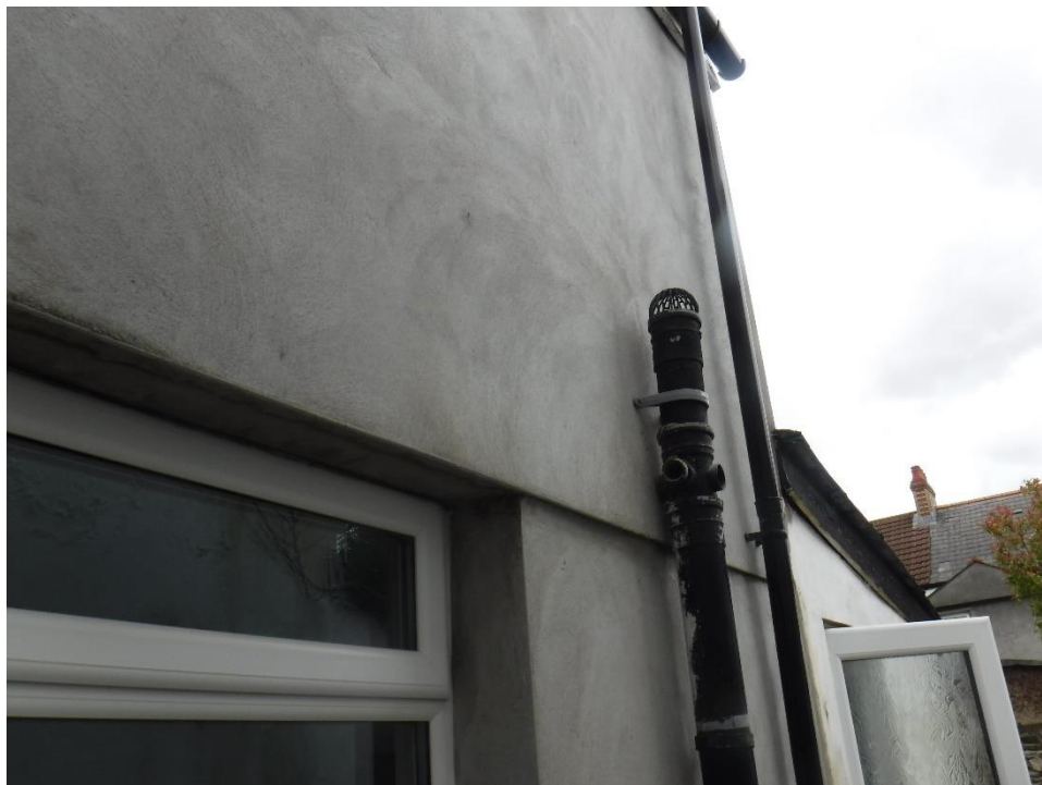
Photograph 11: Exterior - the soil vent pipe is adjacent to the window
