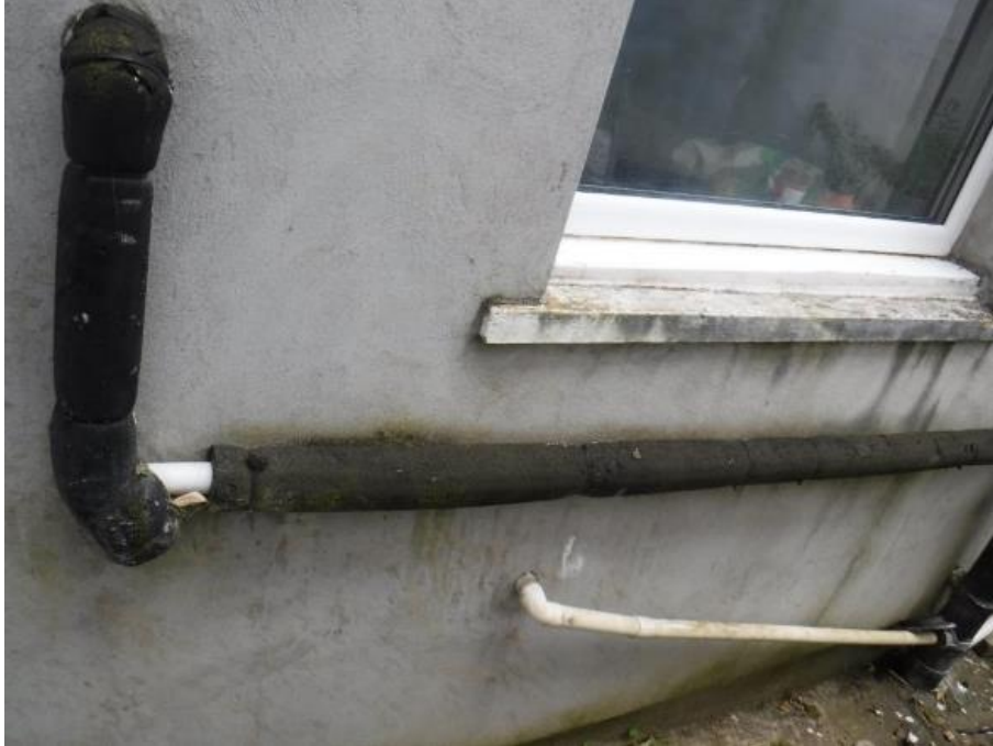
Photograph 9: Exterior - condensate pipe – failed lagging
