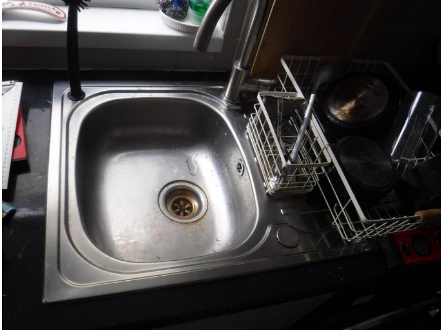
Photograph 43: Minor sealant repair required around kitchen sink
