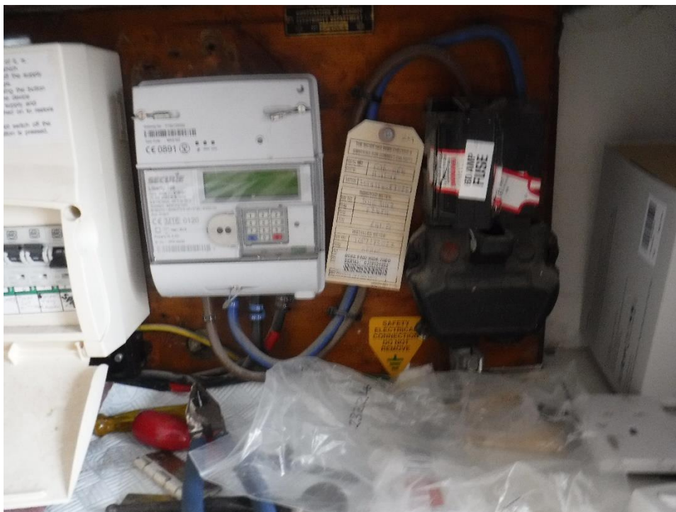
Photograph 50: Meter and service head
