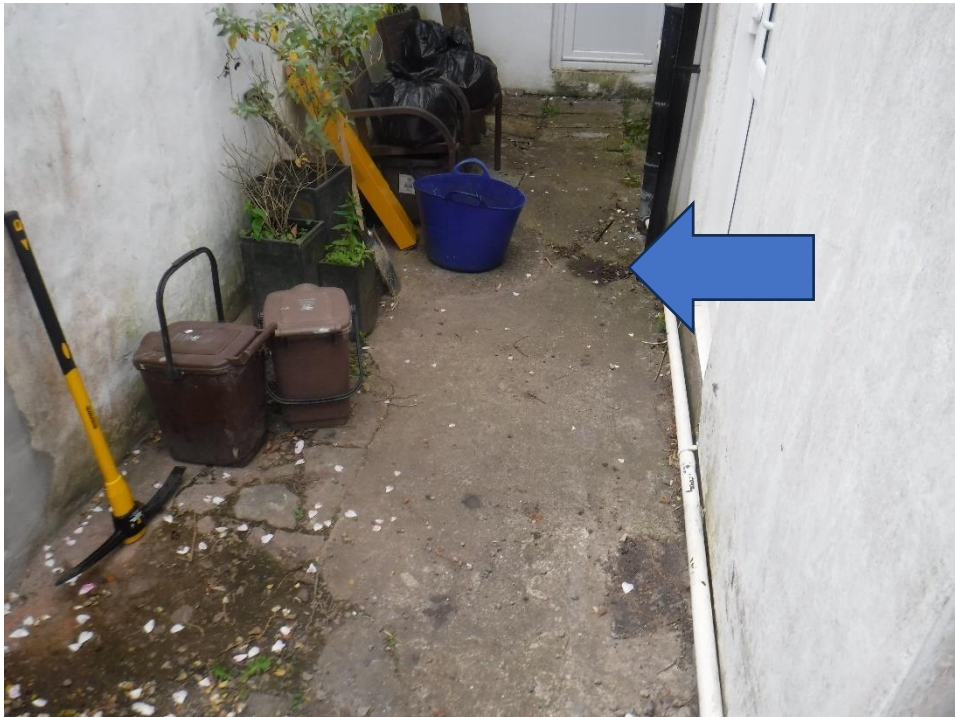
Photograph 10: Exterior - fall to rear (drain inlet location highlighted)
