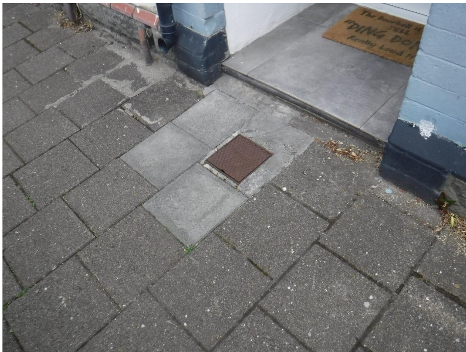
Photograph 51: Location of external stop tap
