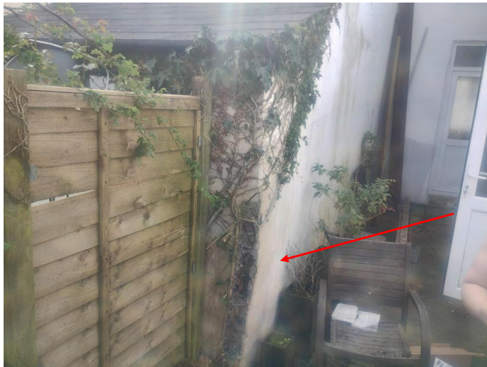
Photograph 60: Garden south boundary wall – extension bulge
