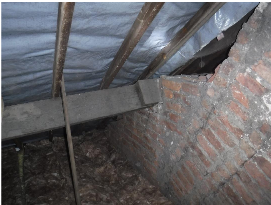
Photograph 19: Roof space - purlins – supported by the party walls
