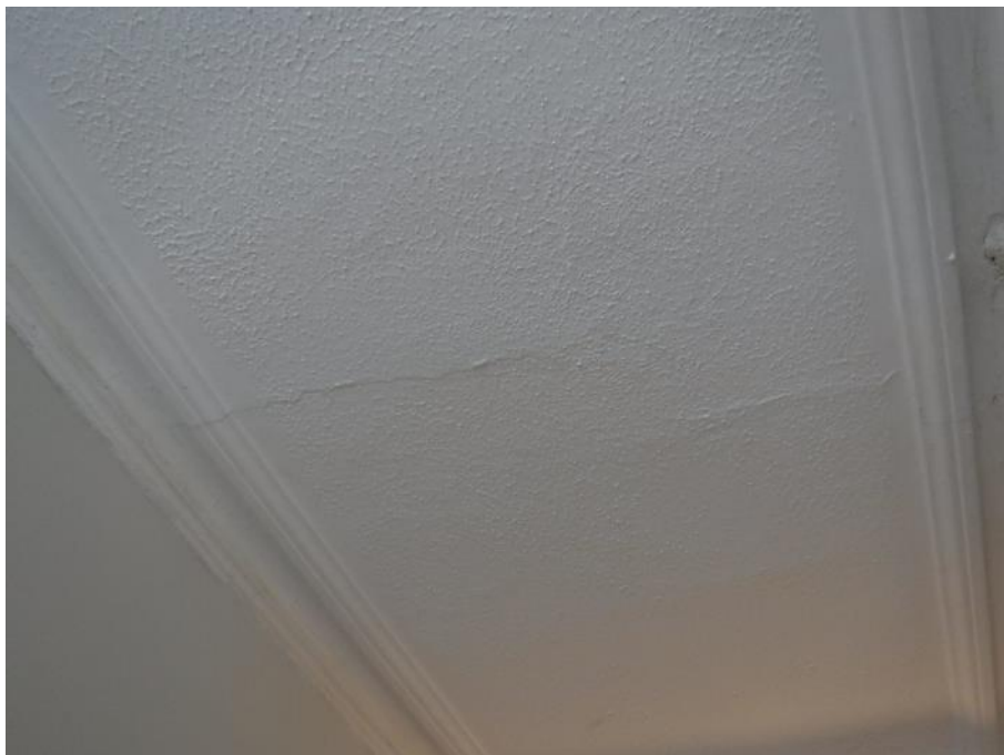
Photograph 27: Hallway - artex ceiling and minor cracking
