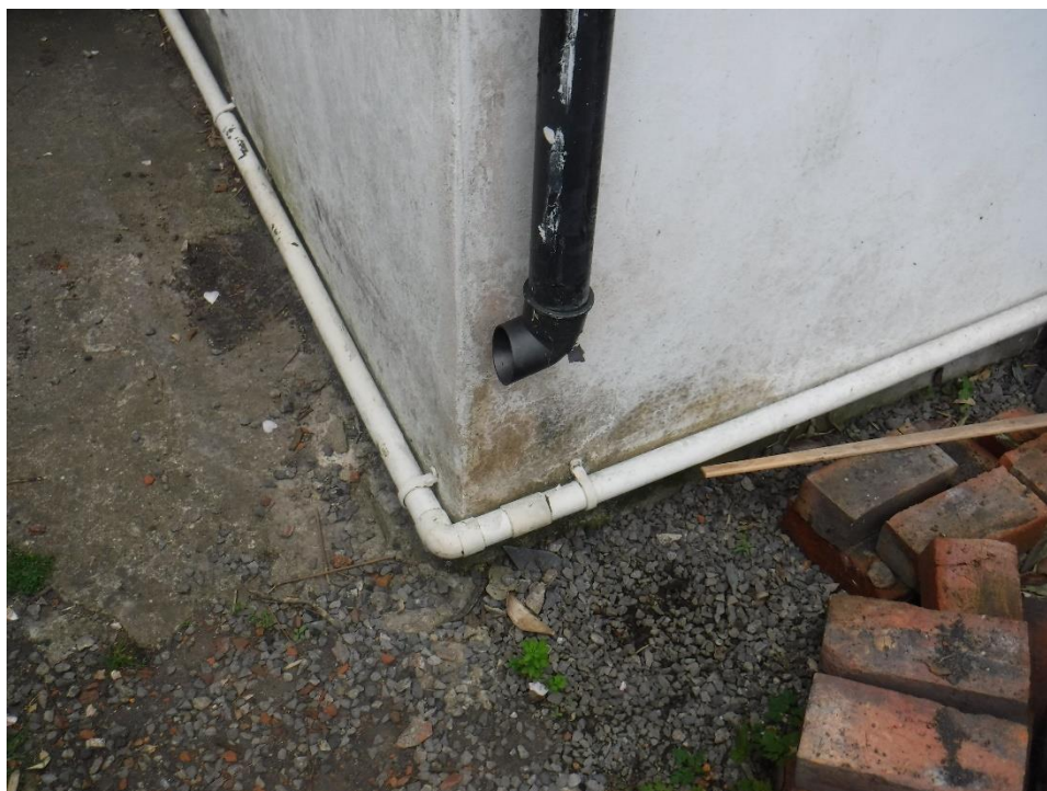
Photograph 8: ...which in turn dispels onto the ground at the rear of the property (inclined towards the sitting room)
