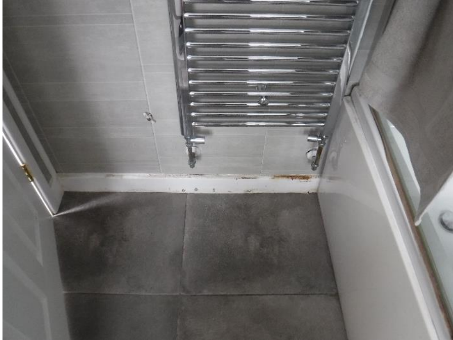
Photograph 53: Bathroom radiator – staining/rot to skirting board
