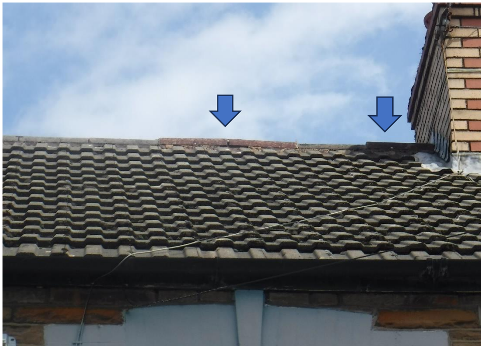
Photograph 6: Roof - several ridge tiles require re-bedding
