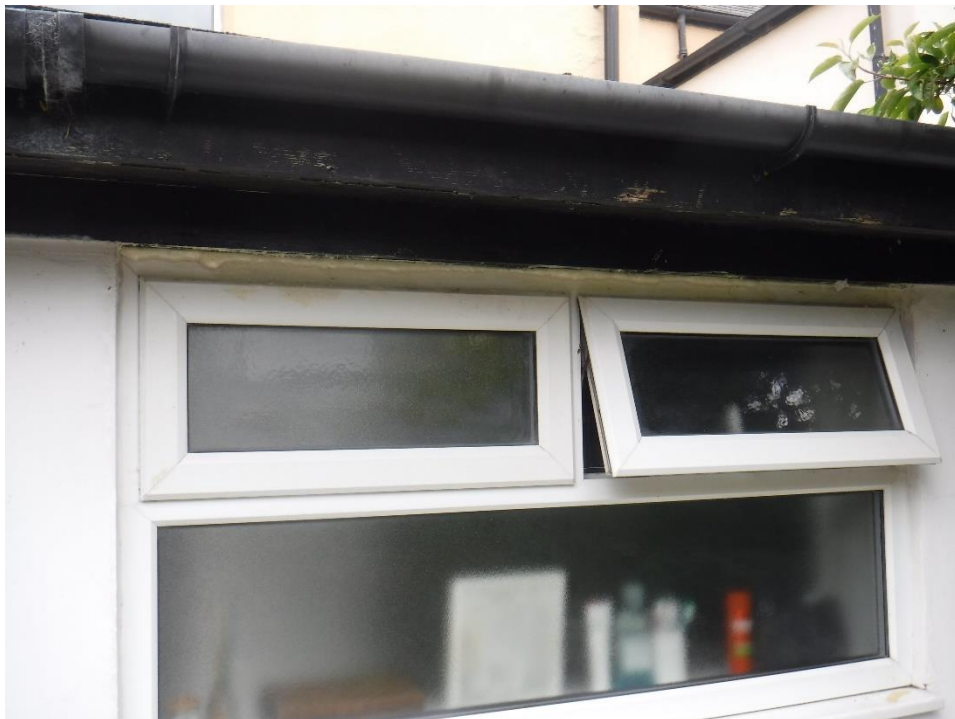
Photograph 16: Bathroom missing upper trim/expanding foam still present
