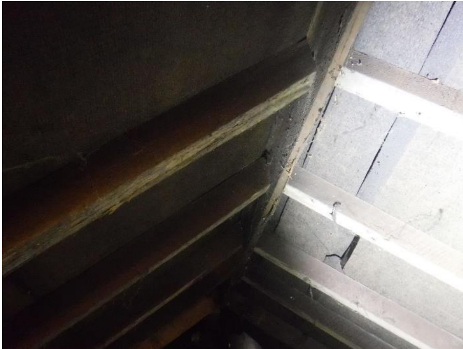
Photograph 39: Roof space - ridge board in fair condition
