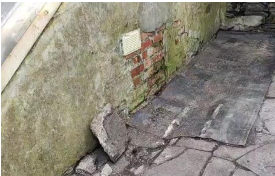
Photograph 8: approximately 1.5m 2 of render was missing to this location and would require a patch repair
