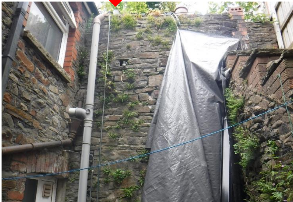
Photograph 14: Soil pipe missing cap/close too window
