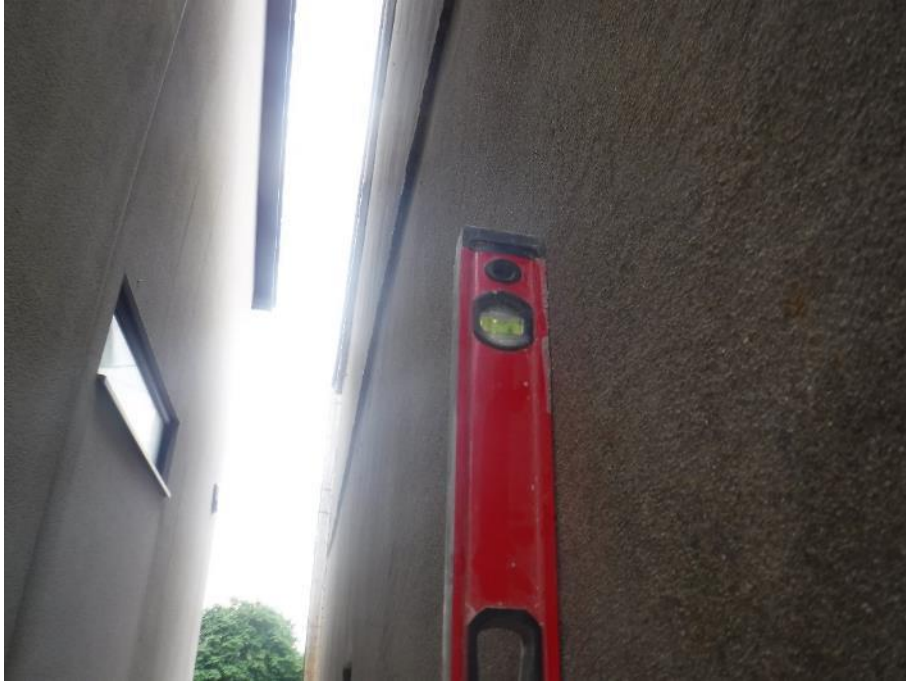
Photograph 17: No significant alignment defects noted
