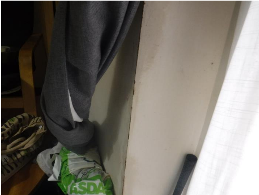
Photograph 55: Corroded angle bead to the dining room, indicative of damp inside the property
