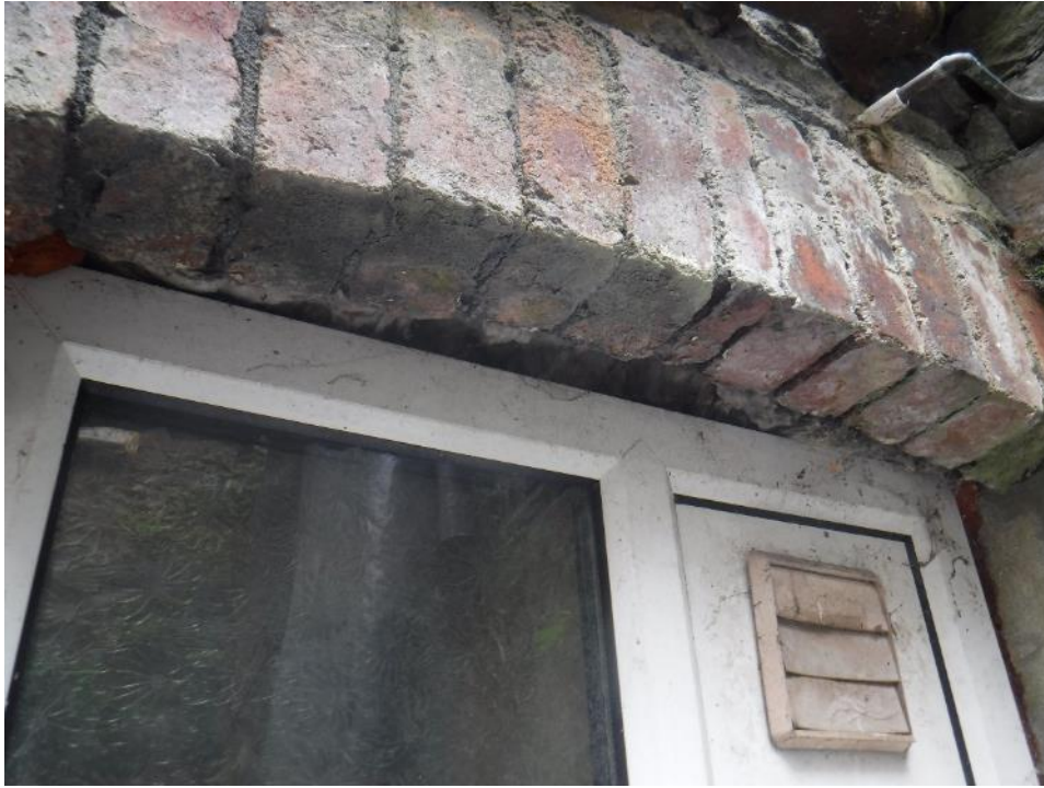
Photograph 21: Spalling and heavy efflorescence to rear lower lintel arch
