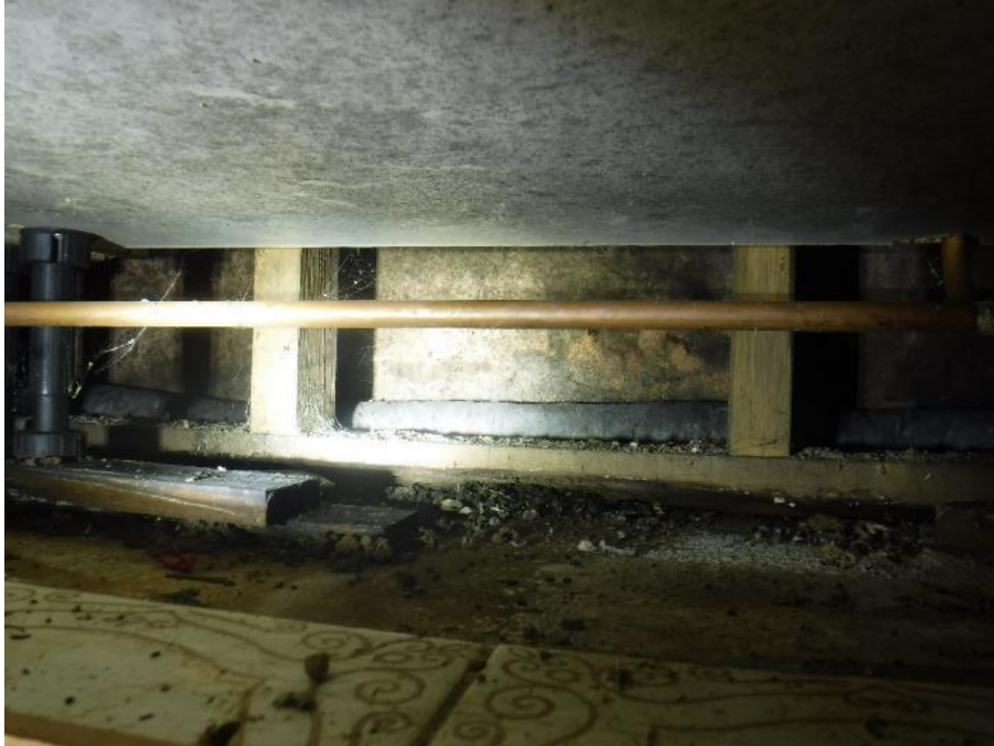
Photograph 59: Kitchen - damp was noted to the kitchen rear wall, note damp proof membrane (presumed) laid above concrete subfloor.
