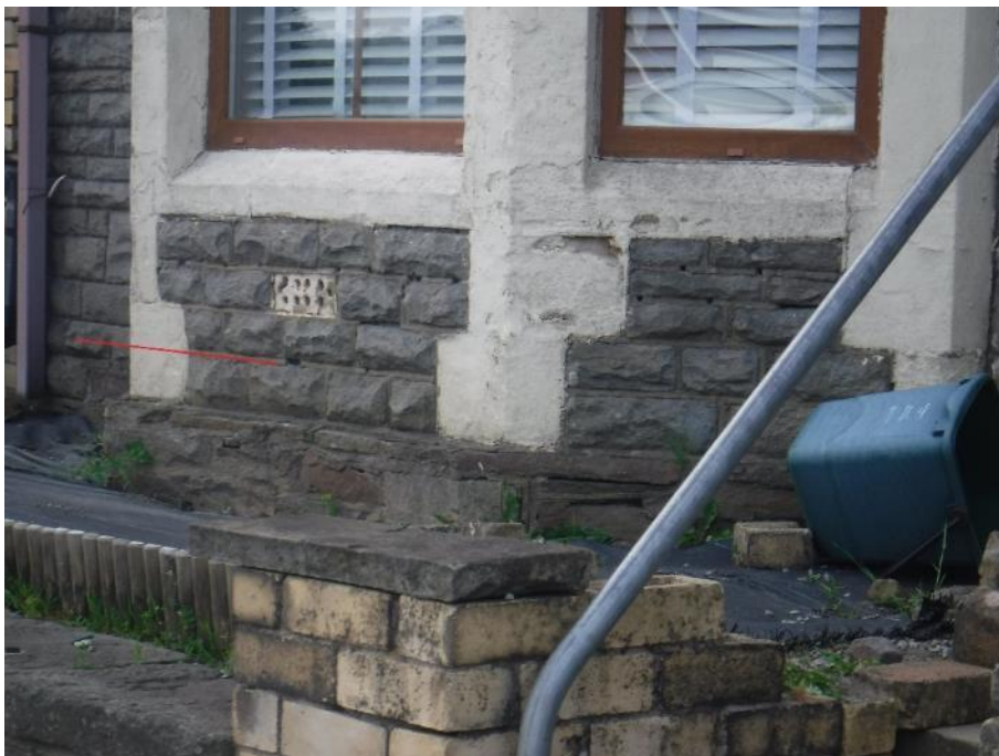
Photograph 24: When compared to the neighbouring property where the plinth course is still visible (line added):
