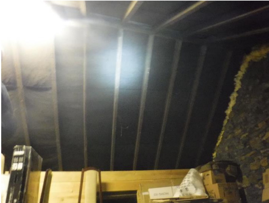
Photograph 41: Roof space - Sarking noted in fair condition overall
