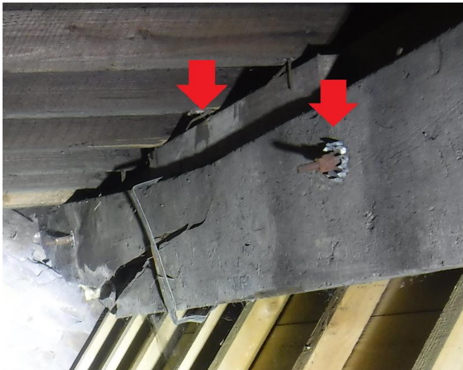
Photograph 34: Purlins sistered up (reinforced) to new supporting member (note dogtooth bolt)
