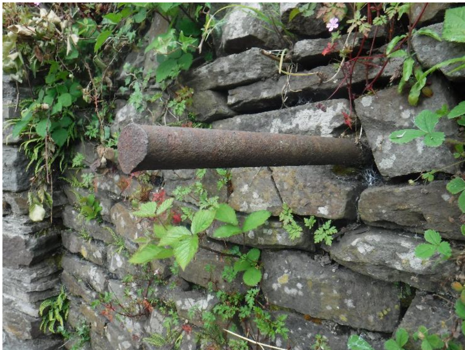
Photograph 86: Tie bar to upper patio garden retaining wall
