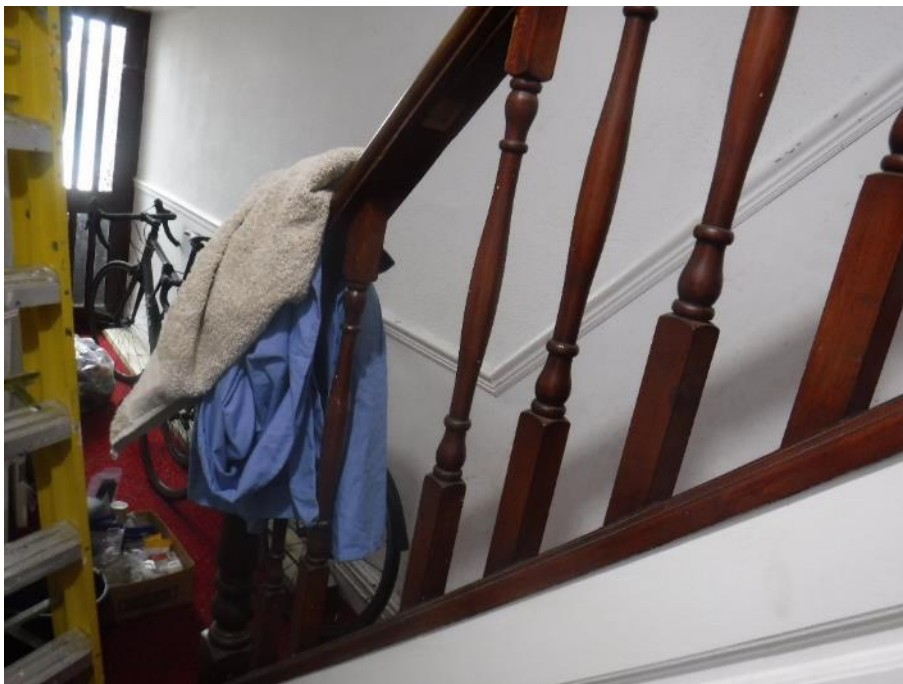
Photograph 70: Spindle missing to staircase (remainder of staircase in fair condition)
