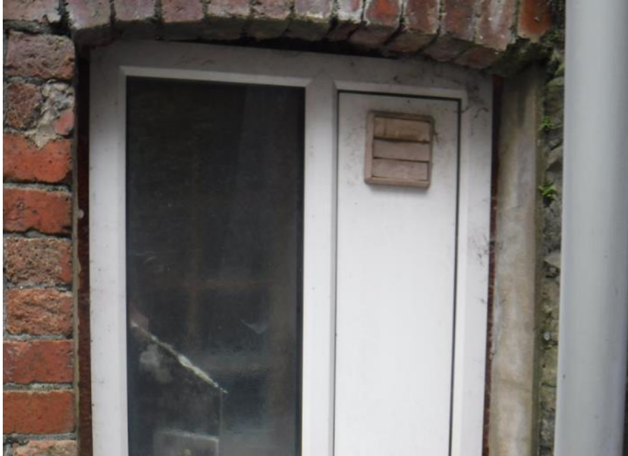
Photograph 29: Far kitchen window requires sealing down the edges with uPVC window trim and silicone
