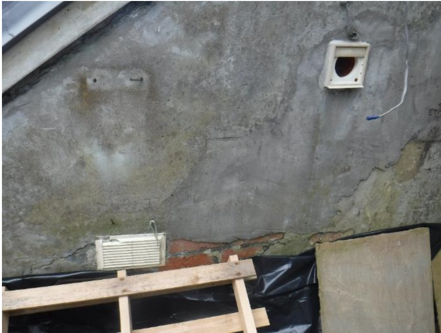
Photograph 7: The gable end in this location requires re-rendering/repairing. There is some ventilation in this area (for the roof) however the fan is not operational.
