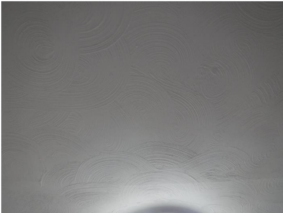
Photograph 48: Artex ceiling in bathroom
