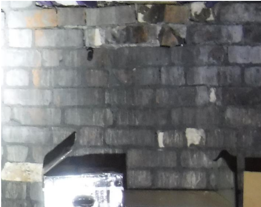
Photograph 45: Roof space - areas of mortar repairs noted
