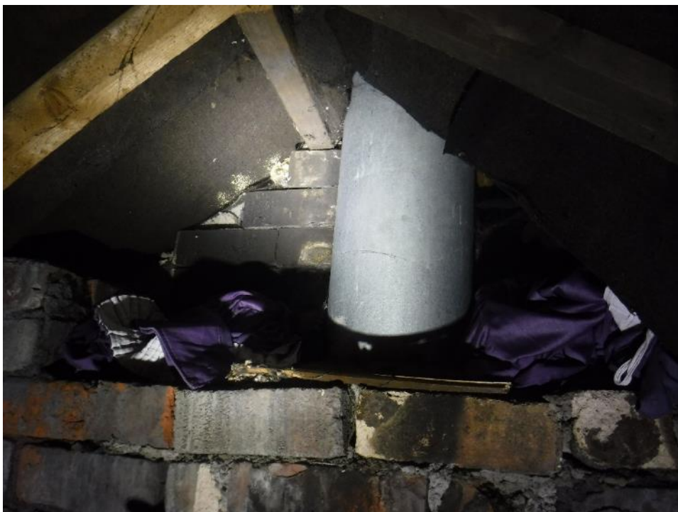
Photograph 44: Roof space – flue/chimney – not compartmentalised with combustibles around it
