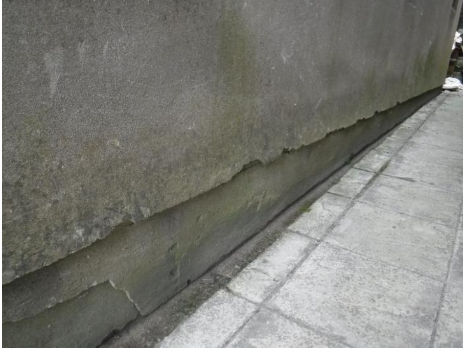
Photograph 15: Cement render to the bottom of the east elevation (we would recommend 150-200mm removal)
