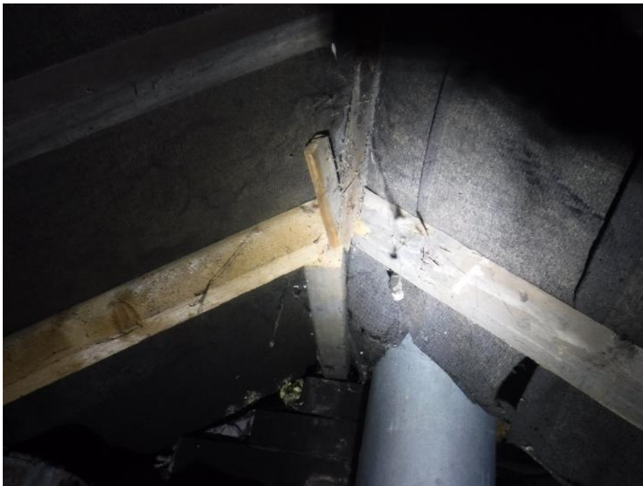
Photograph 40: Roof space – the newly added ridgeboard extension is off centre
