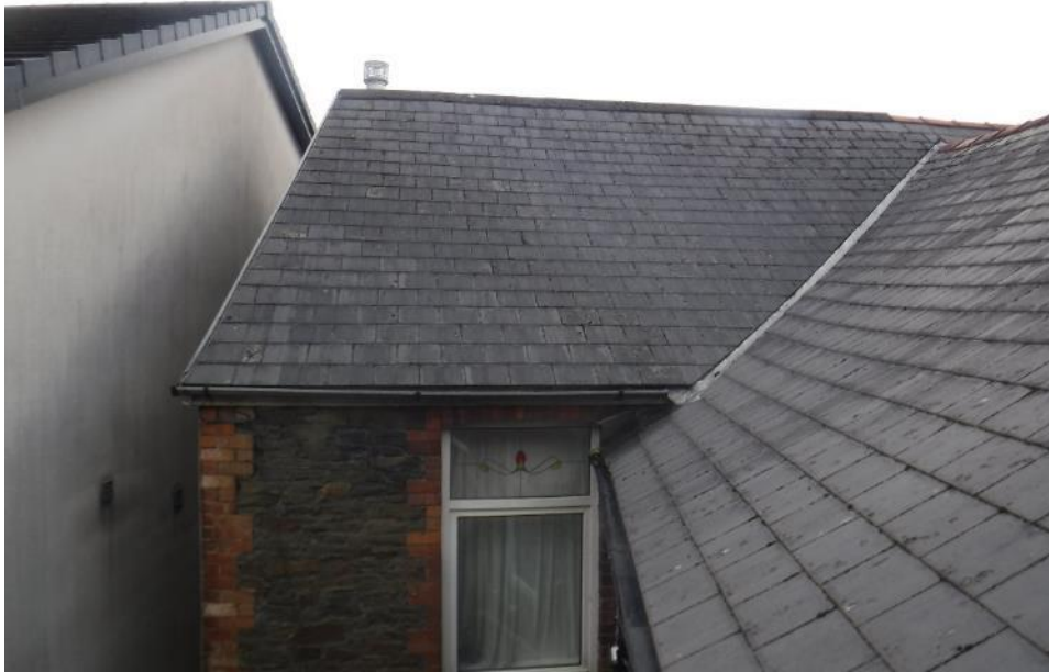
Photograph 5: Rear chimney – removed and roof intact
