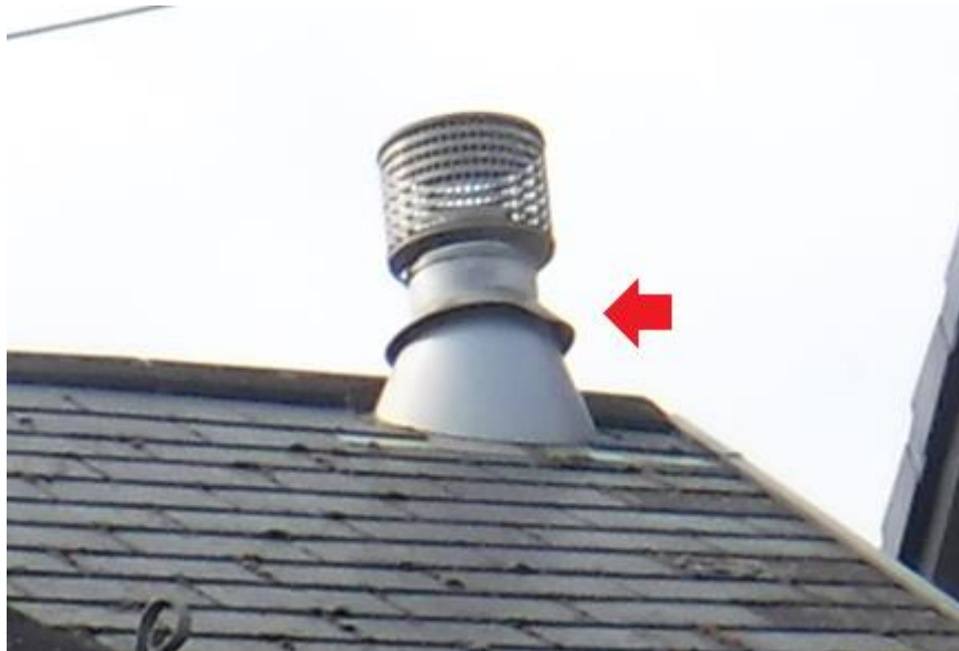
Photograph 4: Front chimney – minor dent observed
