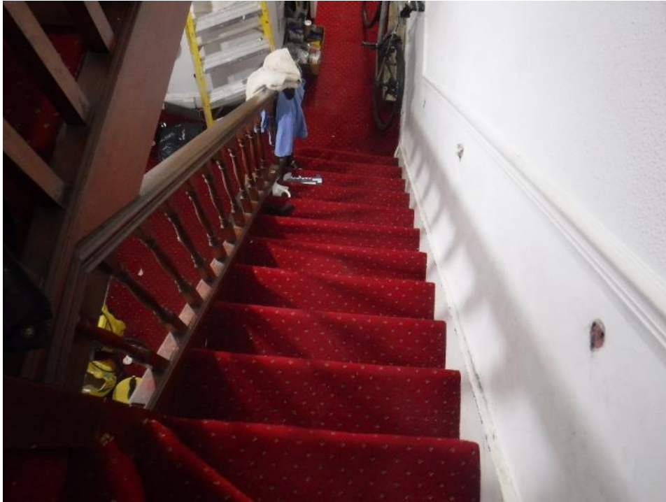
Photograph 69: The staircase was covered (restricting examination) however it was noted as level, no significant creaking on heel tests and the stringer was in good order (note patch repairs to wall)
