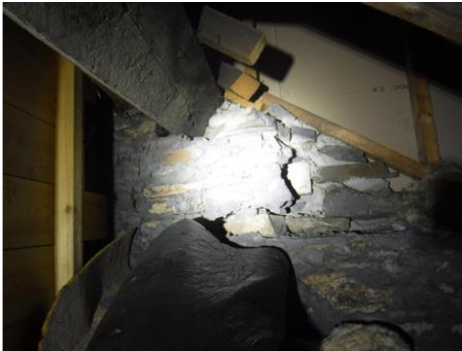
Photograph 38: Roof space - gap/un-mortared section of wall (note proximity to purlin) at the NW
