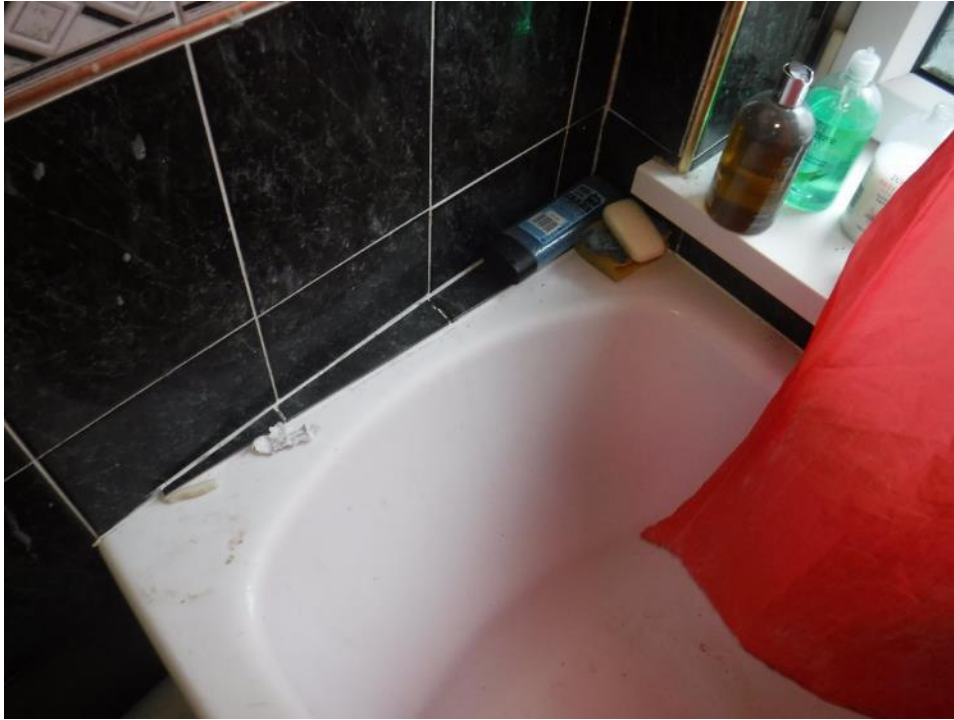
Photograph 71: Bathroom – sealant degraded
