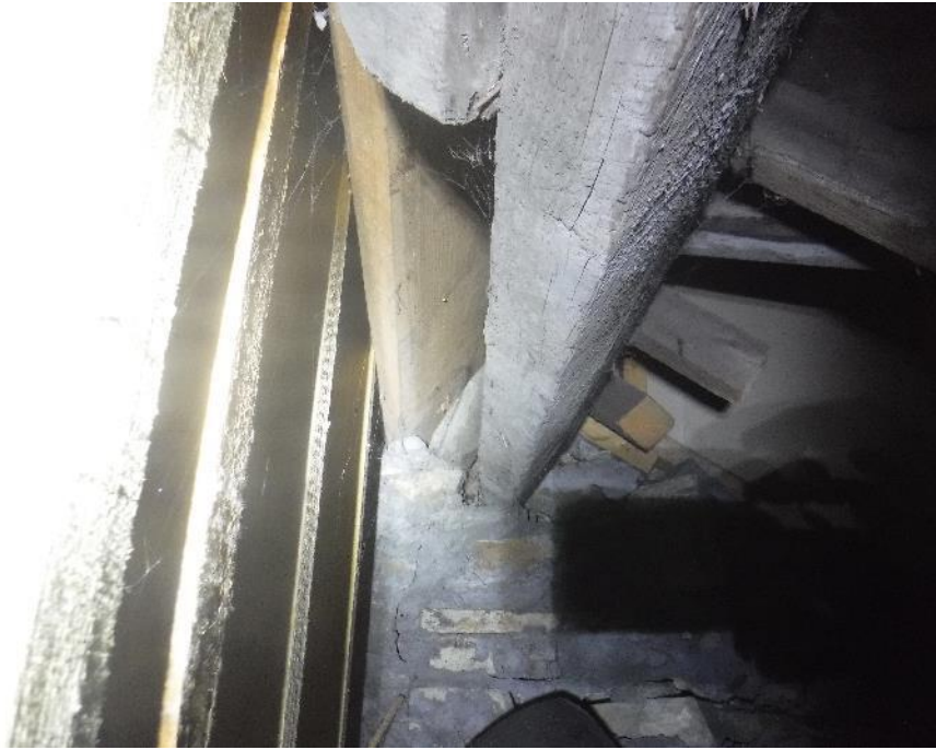
Photograph 37: Roof space - external view of cracked purlin location (no sagging noted)
