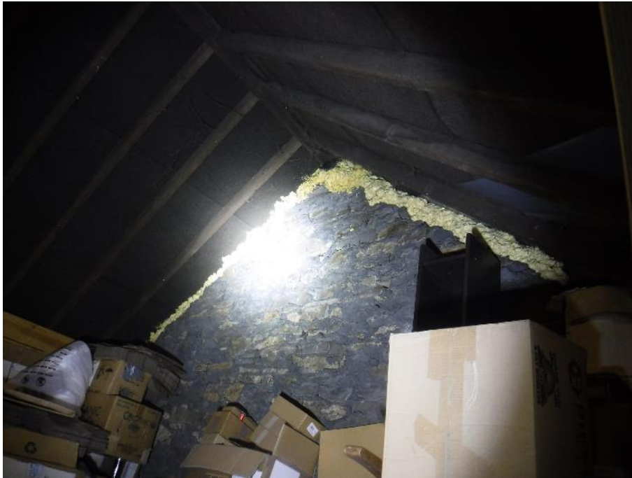
Photograph 43: Roof space - Expanding foam was found up to the rafters in both walls. Not believed to be fireproof expanding foam (which has pink colourants)
