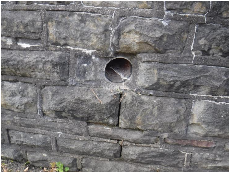
Photograph 92: Retaining wall to front of property - weephole
