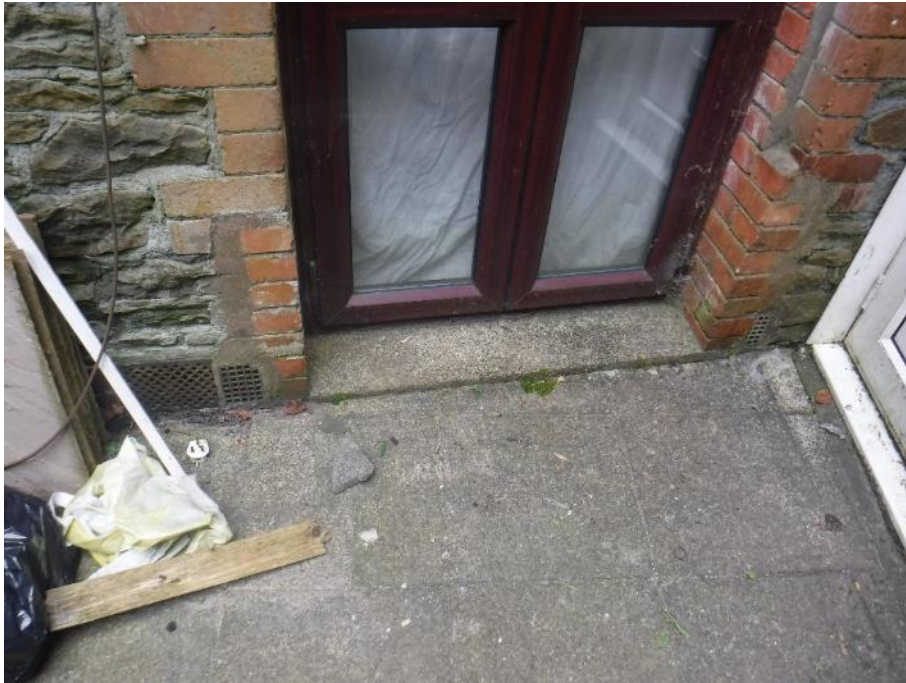
Photograph 25: Three airbricks were noted to the exterior of the property at ground level, believed to pass air downwards to the sub-floor void
