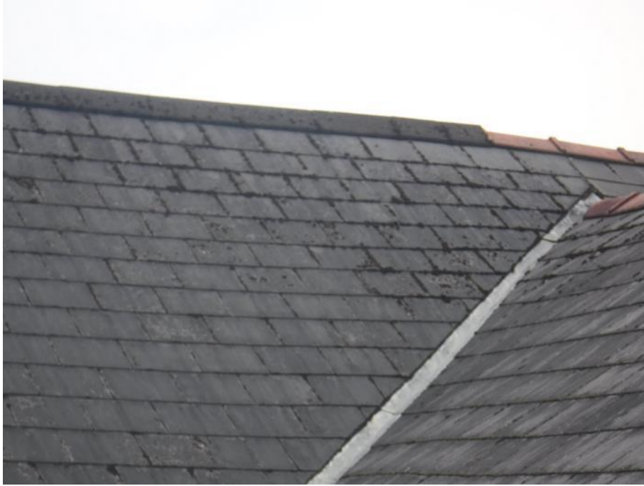
Photograph 9: Valleys noted in fair condition, also please noted 3m2 moss growth (presumed to be unreachable area without increased access)
