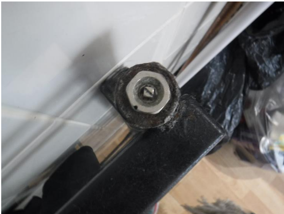
Photograph 74: Bathroom – corrosion to radiator
