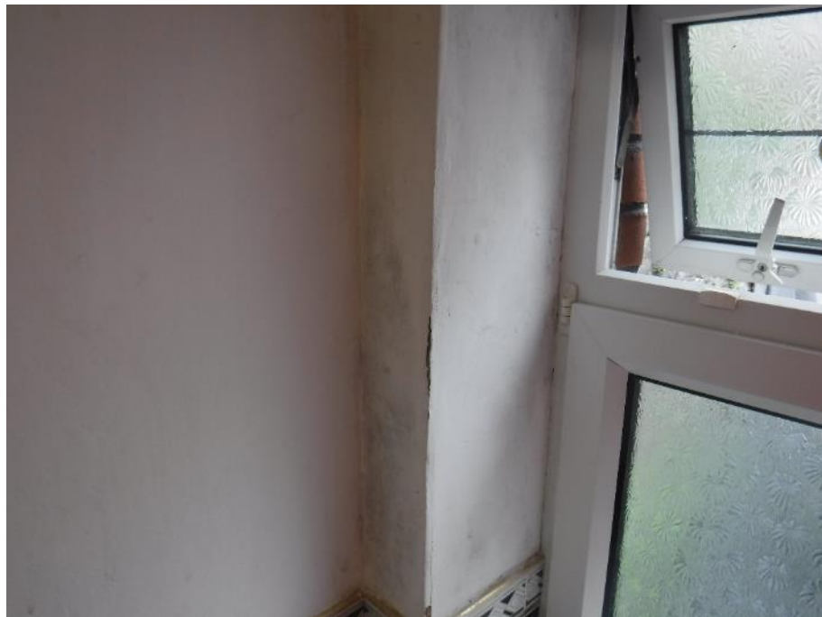
Photograph 54: Corroded angle bead to bathroom
