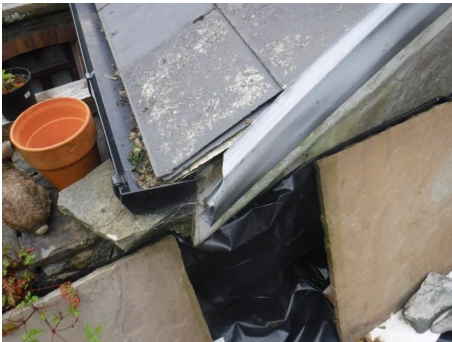
Photograph 6: Extension roof corner - dry-verge had a minor detachment to the east and requires re-attaching, also the guttering require re-attaching
