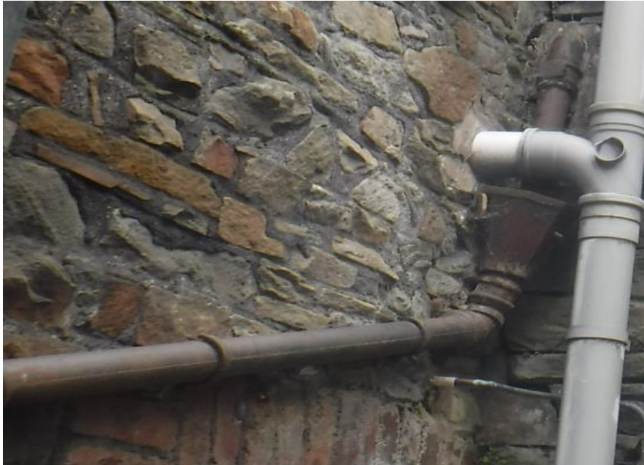
Photograph 13: Cast iron drainage
