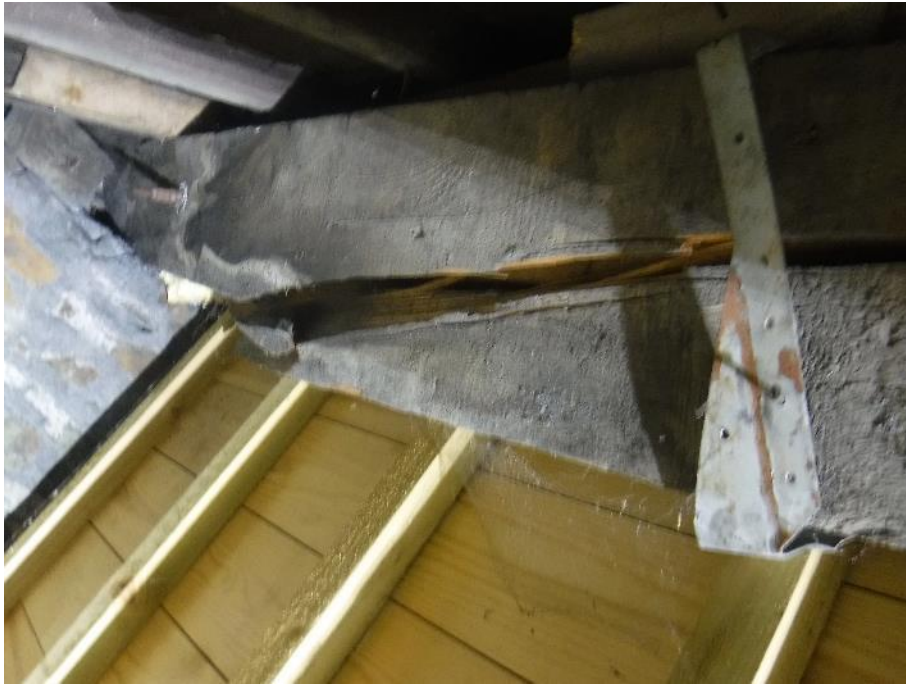
Photograph 33: Further view of crack to purlin
