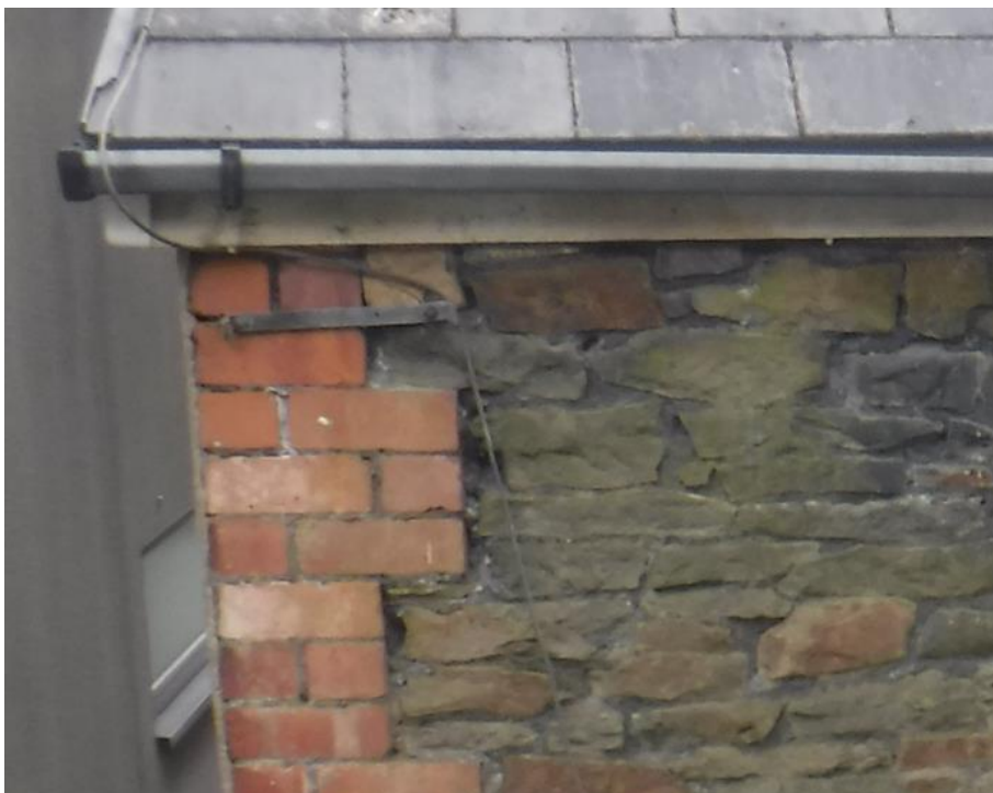
Photograph 26: Areas of mortar loss noted
