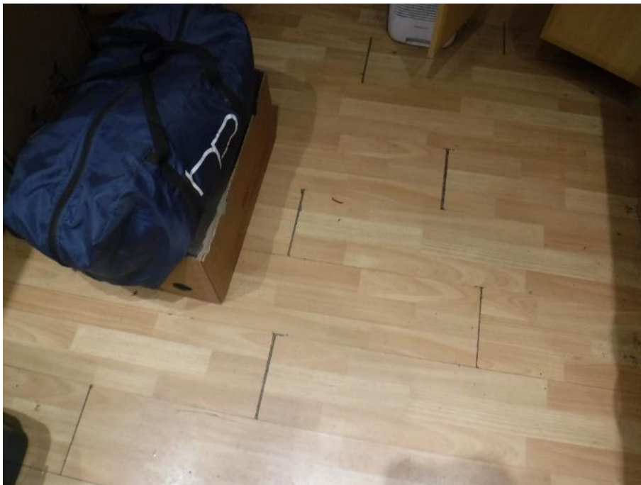
Photograph 60: Kitchen - the laminate flooring was degrading and would require replacement in the short-medium term
