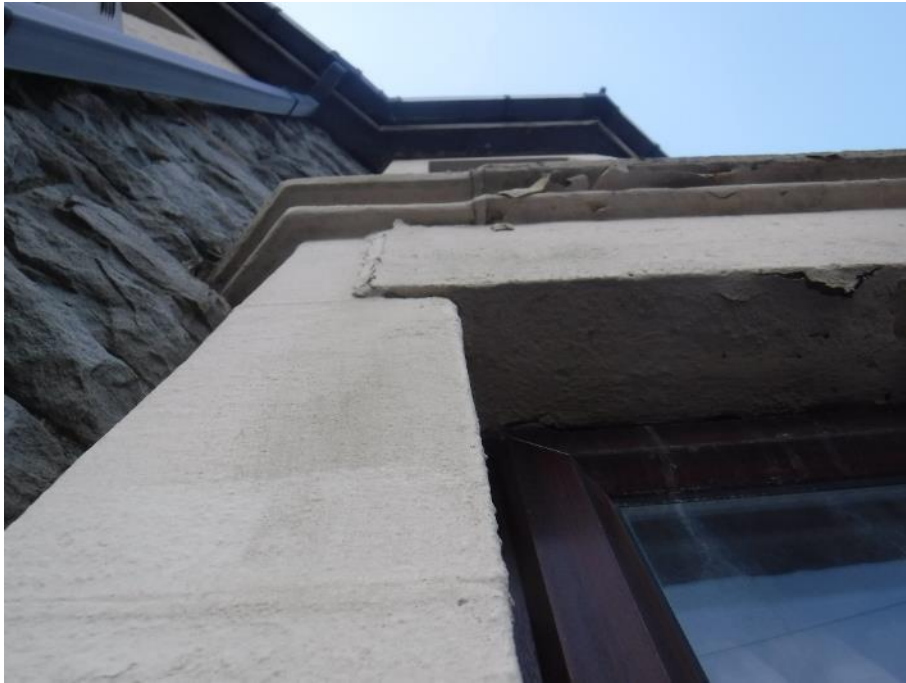
Photograph 19: Alignment defect to bay window jambs/lintels at west
