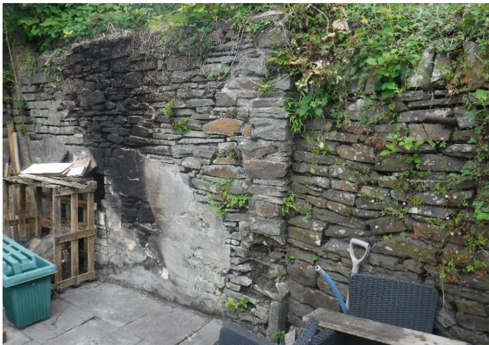
Photograph 84: Further retaining wall to upper patio garden area - supporting upper garden
