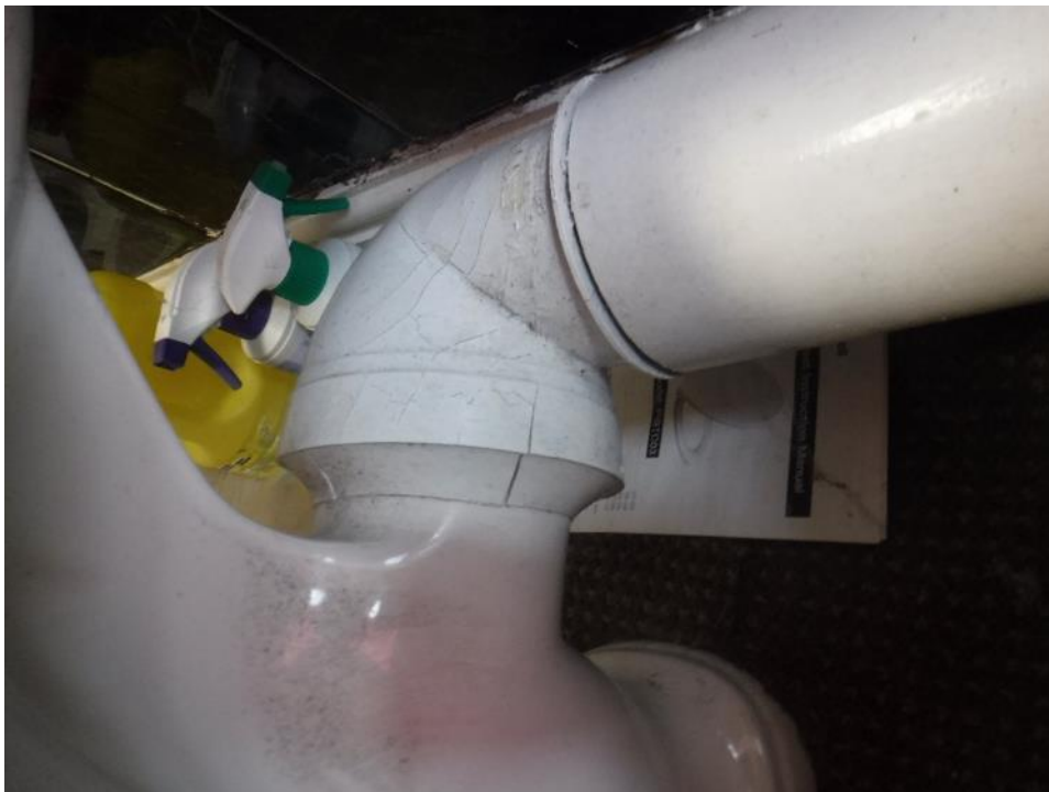
Photograph 72: Bathroom – crack in soil pipe collar
