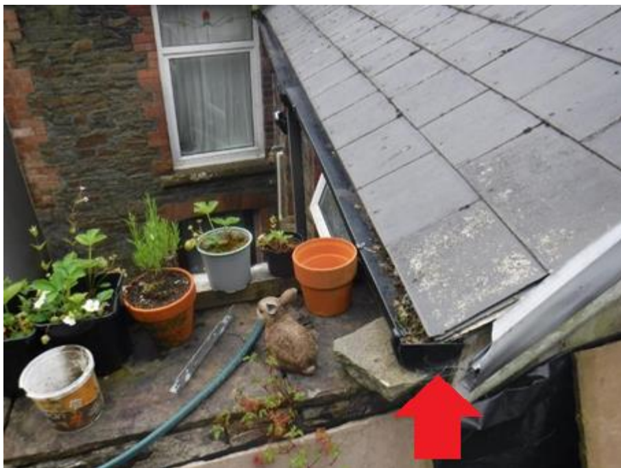
Photograph 12: Further temporary fix to the stop-end
