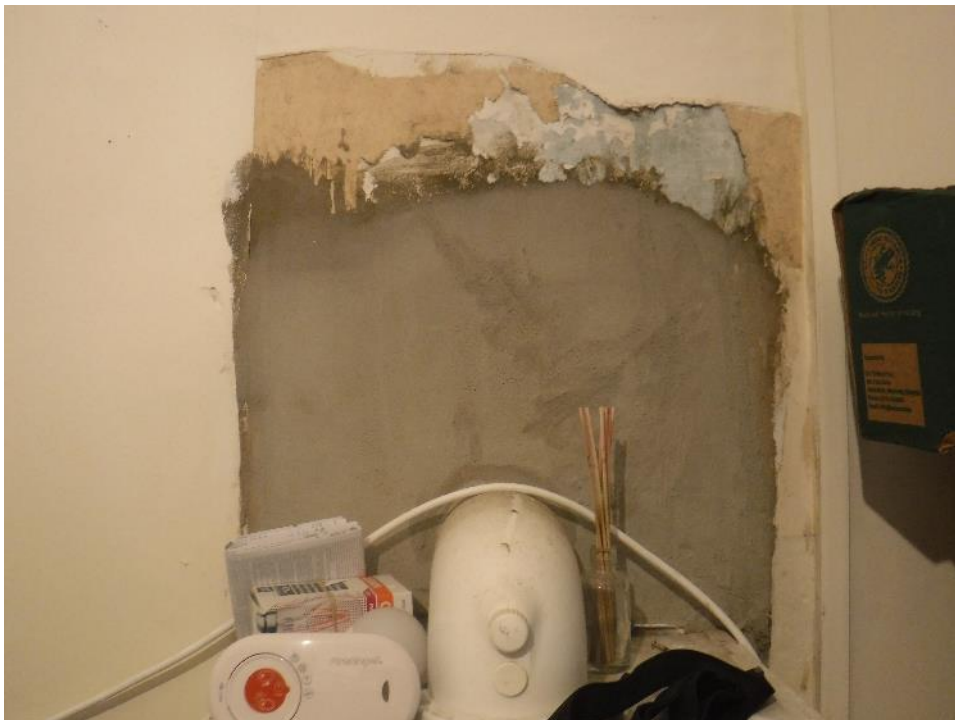
Photograph 58: Walls – boiler installation plaster repair
