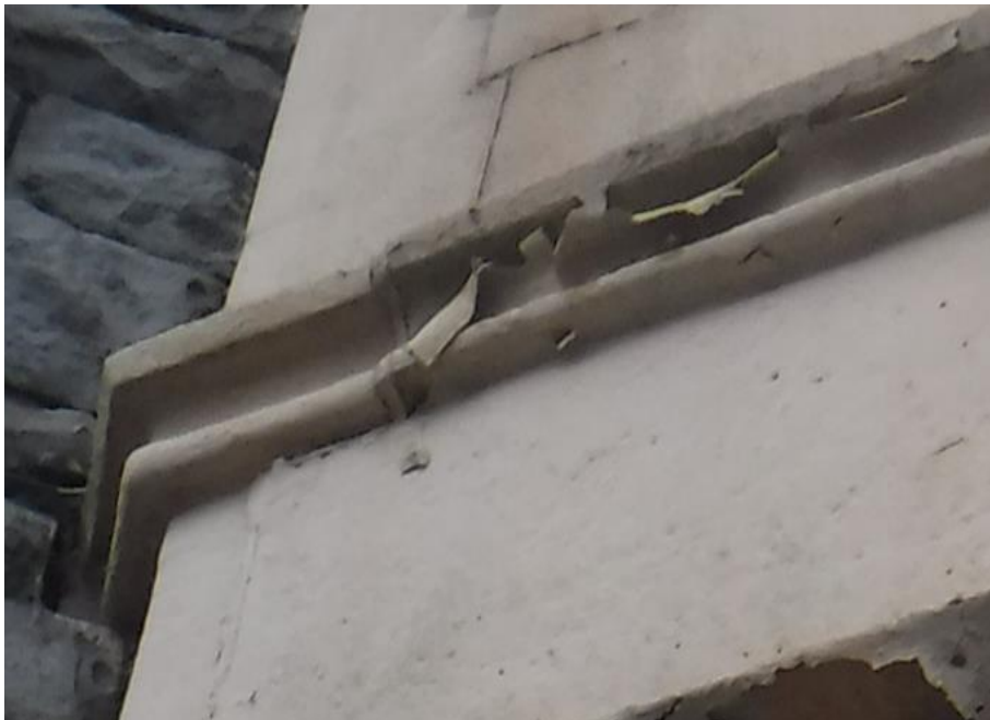
Photograph 18: Alignment defect to bay window jambs/lintels at west (also noted paint condition)
