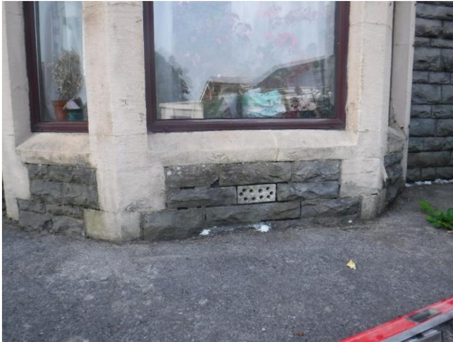
Photograph 23: External ground infilled with concrete to the front elevation, also note single air brick we would recommend installation of more air bricks to this elevation
