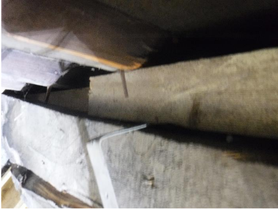
Photograph 35: Roof space - view of sistered purlin
